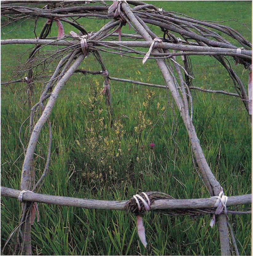
The dome framework of a purification lodge, made from willow branches
