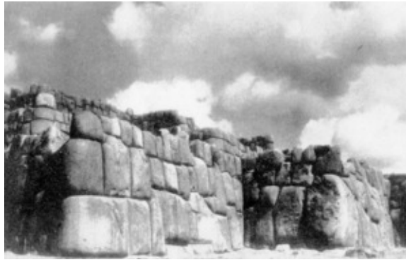
ZIGZAG WALLS AT SACSAYHUAMAN, NEAR CUZCO, PERU (From Heinrich Ubbelohde-Doering, The Art of Ancient Peru , 1952. Courtesy Ernst Wasmuth, Publisher, Tübingen, Germany.)
