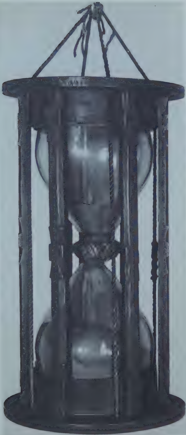
A ship's four-hour sand-clock, probably from the eighteenth century.
