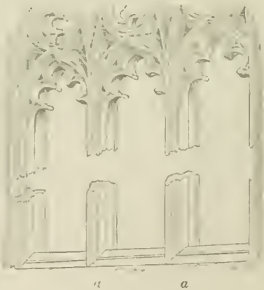
Mullion : Window from Carlisle Cathedral.
