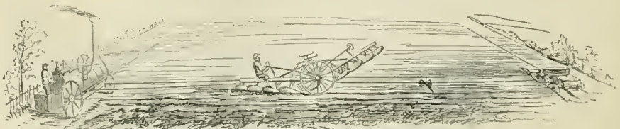
Fig. 12.—Fowler's Anchor, Engine, and Plough at work.
