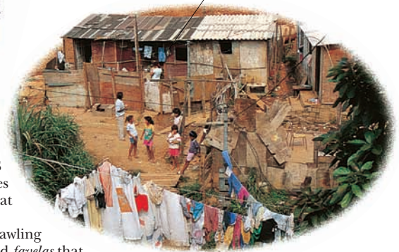
The homes in this shantytown in São Paulo are built from wood and corrugated metal.
