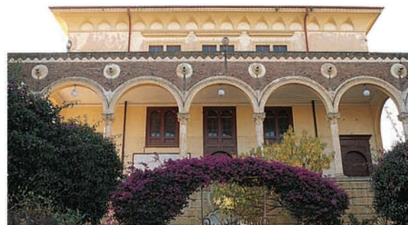
This theater in Asmera, the capital of Eritrea, is an example of the fine Italian-style architecture found in parts of the city. Eritrea was once an Italian colony.
