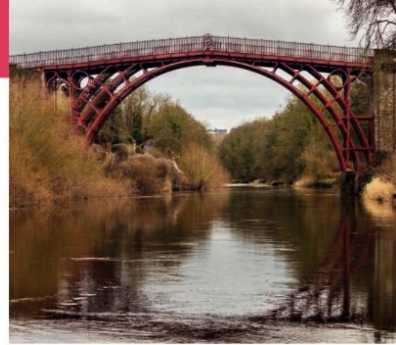
▲ The famous Iron Bridge, opened in 1781. People paid a toll to use it. Before this, bridges were made of wood or stone.
