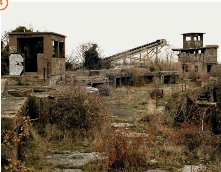
▲ The roof of Cliffe Fort, built in the 1860s to guard the estuary. Now owned by a company that dredges gravel from the river bed.
