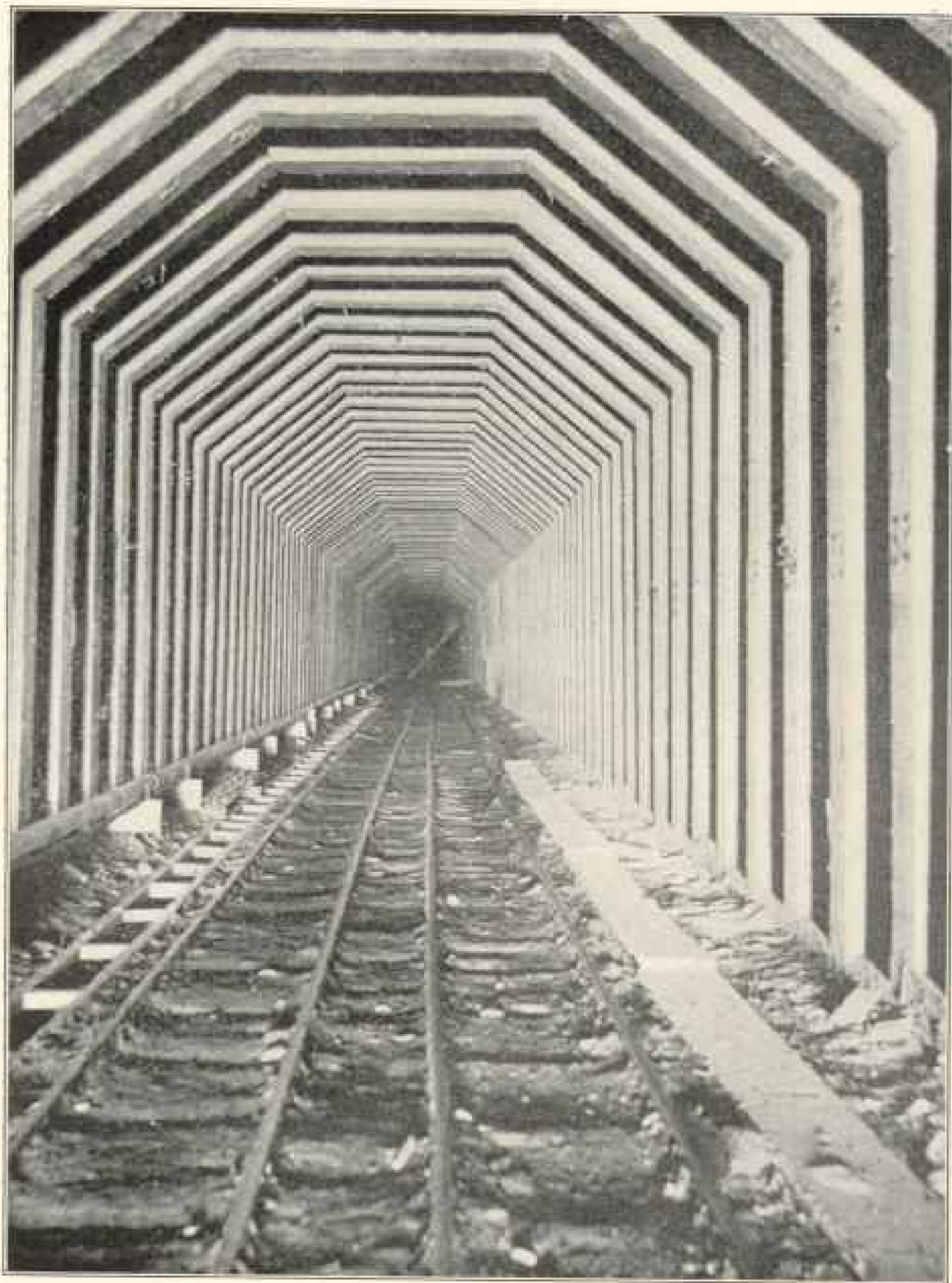
Timbering in the West End of the Gunnison Tunnel.
