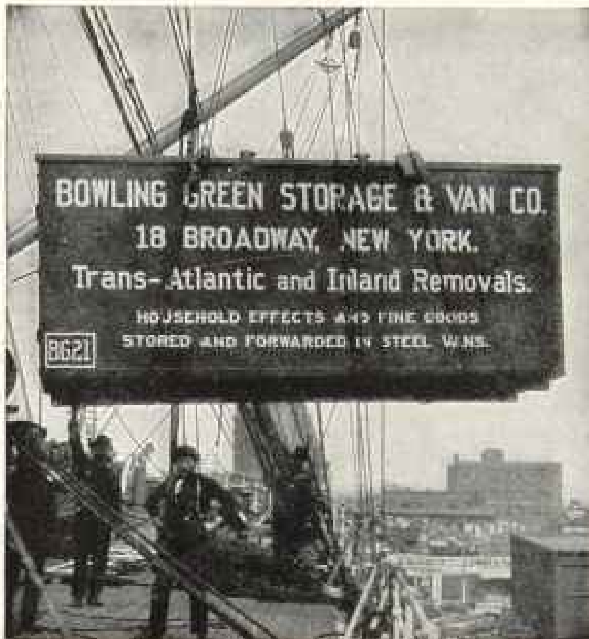
HOISTING LIFT-VAN ON BOARD STEAMSHIP
