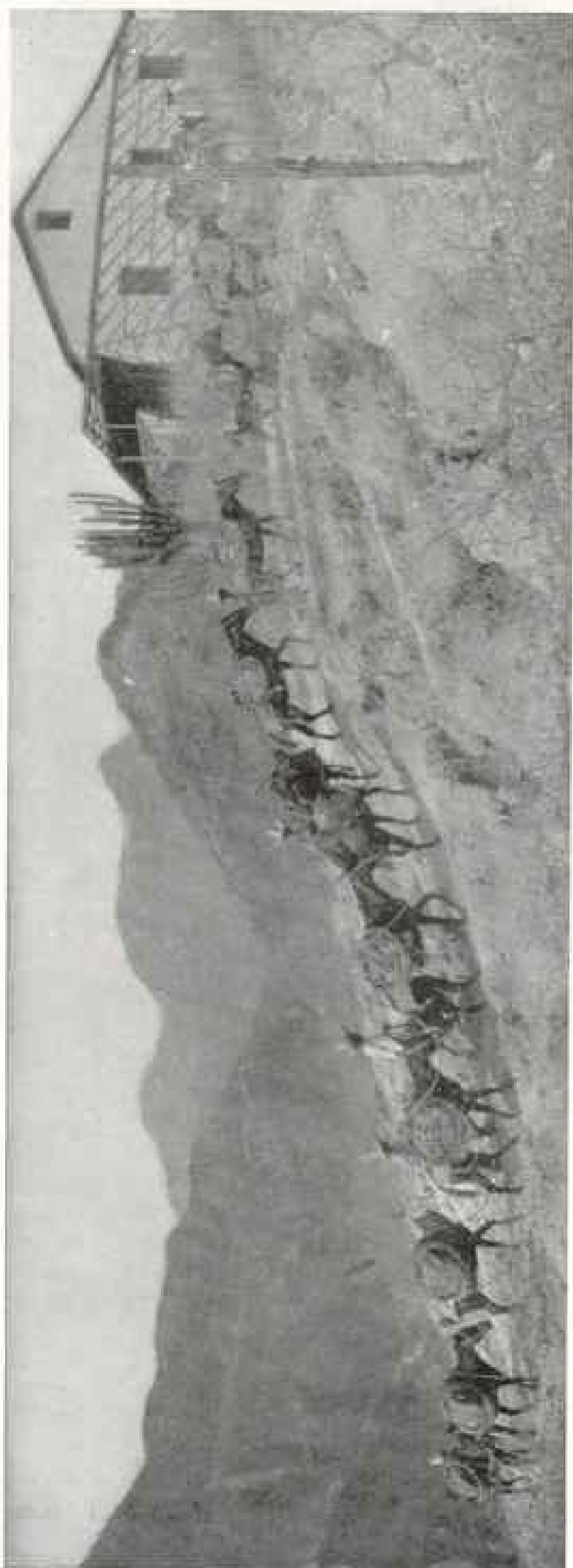
PICTURE 10. CARRYING 2,300 FEET OF \frac{7}{8} STEEL, AÉRIAL TRAMWAY CABLE ON 12 MULES (SEE PAGE 900)
