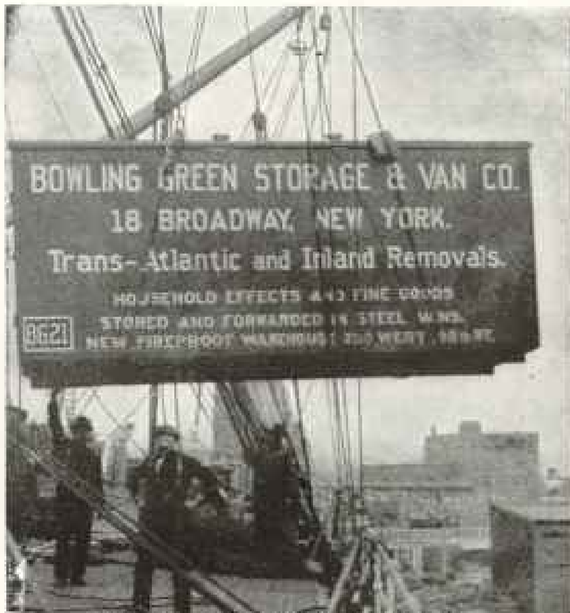
HOISTING LIFT-VAN ON BOARD STEAMSHIP
