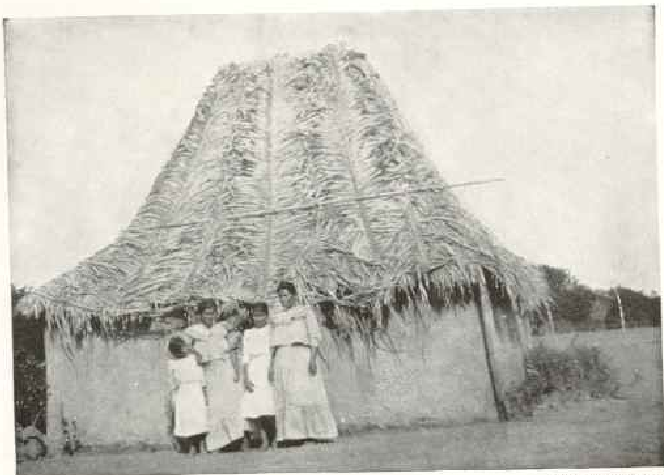
PROVISIONAL, SUMMER ROOF, MADE OF THE LEAVES OF THE NATIVE ROYAL PALM ( Attalea gomphococca ): NOTE THE LONG PALM LEAVES
