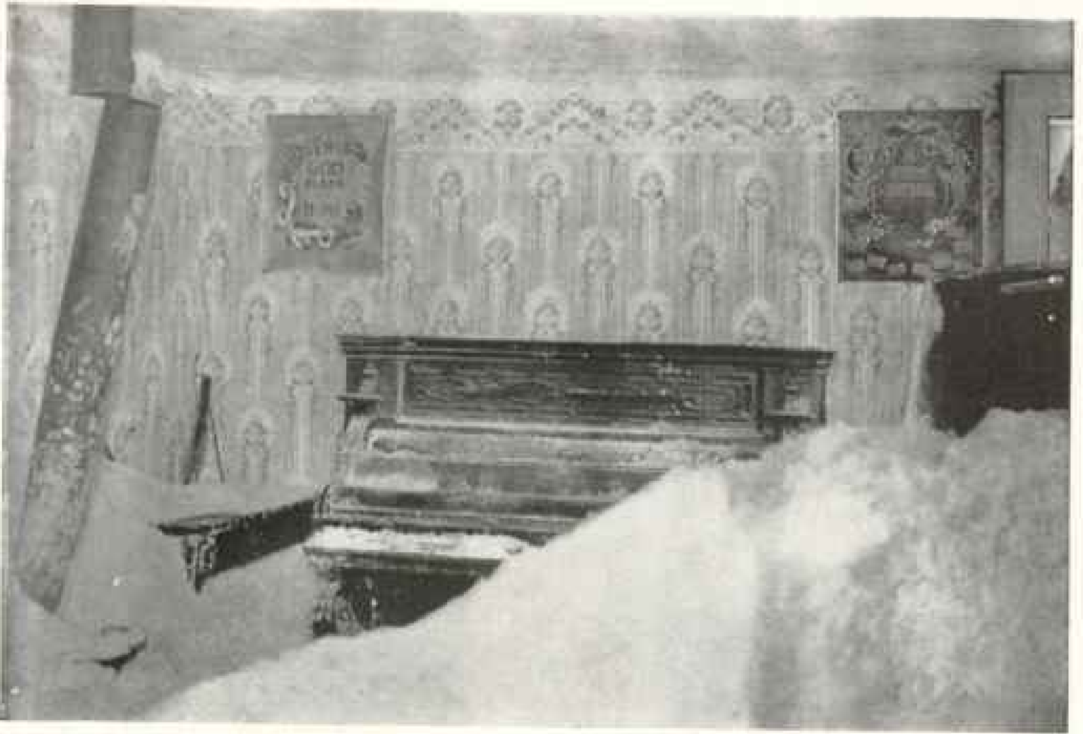
HOUSE AT KADIAK RUINED BY AVALANCHE OF ASHES FROM HILLSIDE. Weight of ashes from hillside avalanche crushed in roof and almost filled the interior of this house. St. Paul, Kadiak, June 9, 1912
