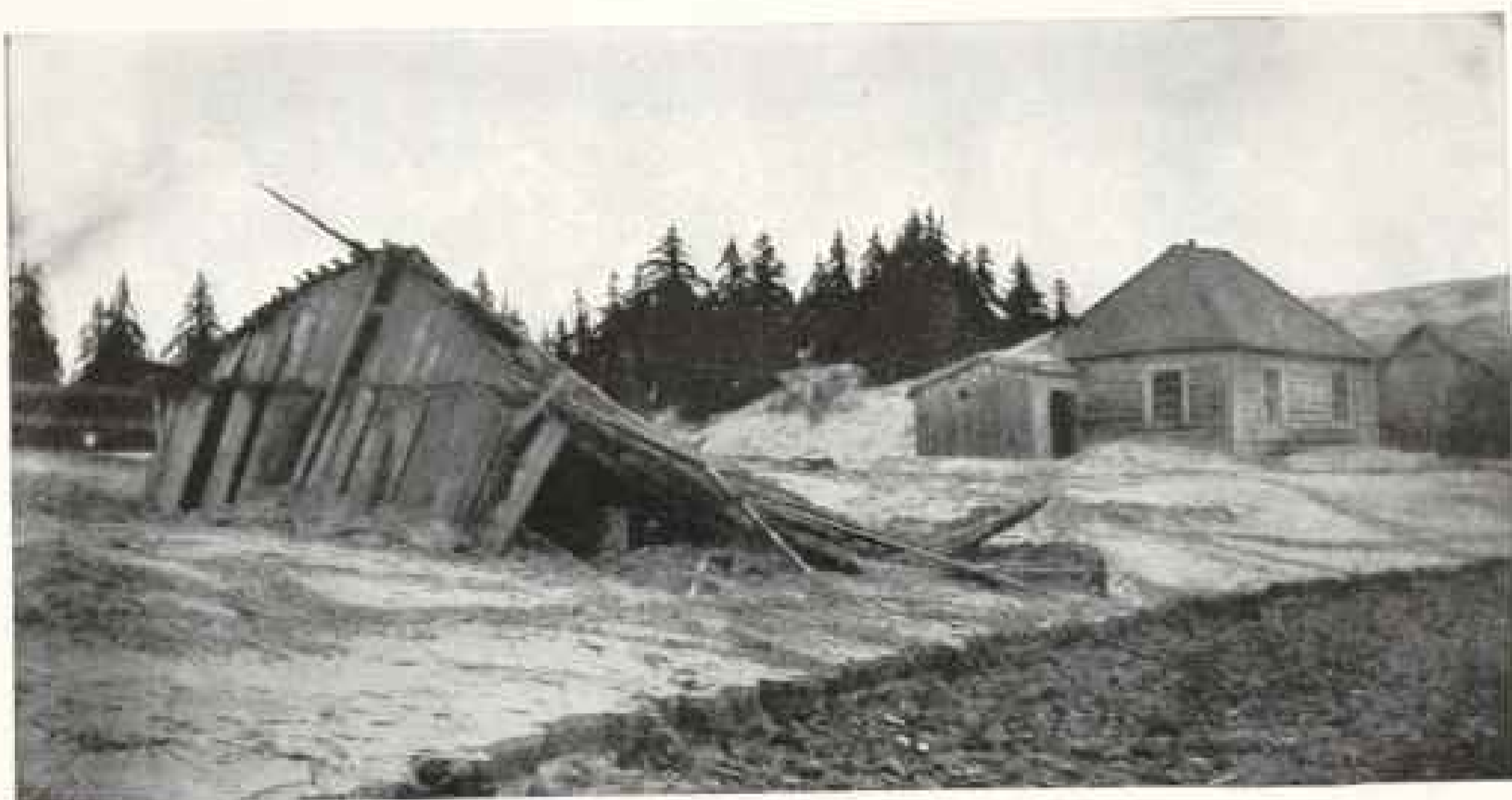
FRAME STRUCTURE CRUSHED BY WEIGHT OF ASHES
