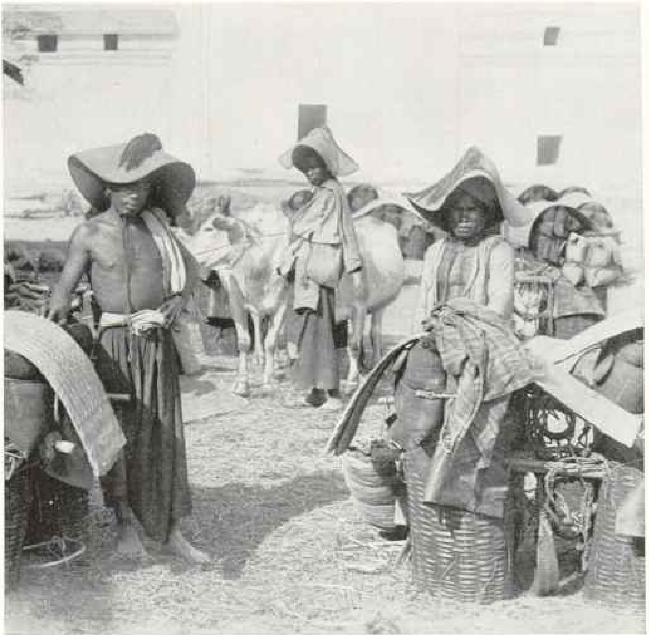
SHANS LOADING COMMISSARIAT STORE
