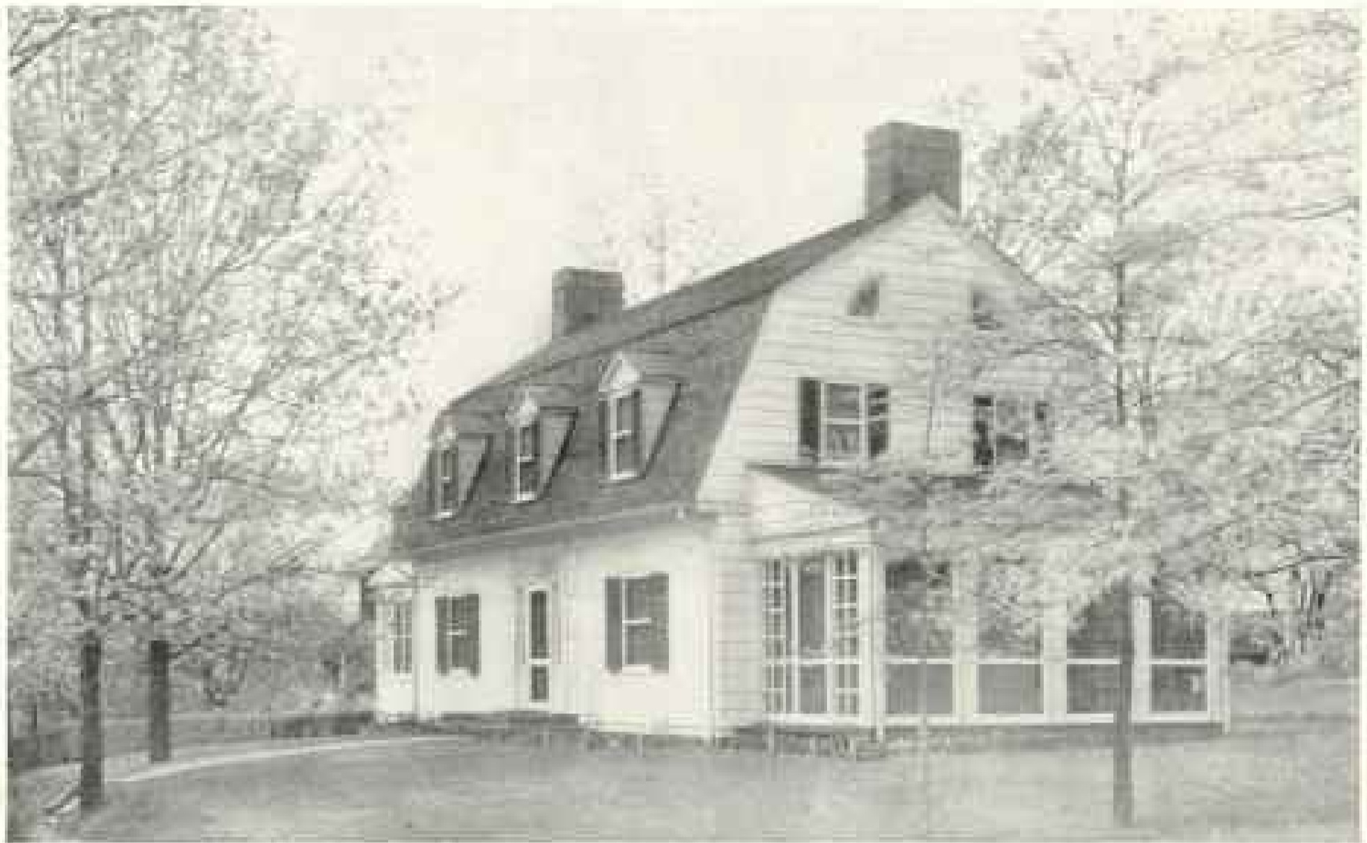
House of Daniel W. Sycr, Esq., Ken Gardens, Long Island, N. Y. Asmar Embury II, Architect, New York, N. Y.
