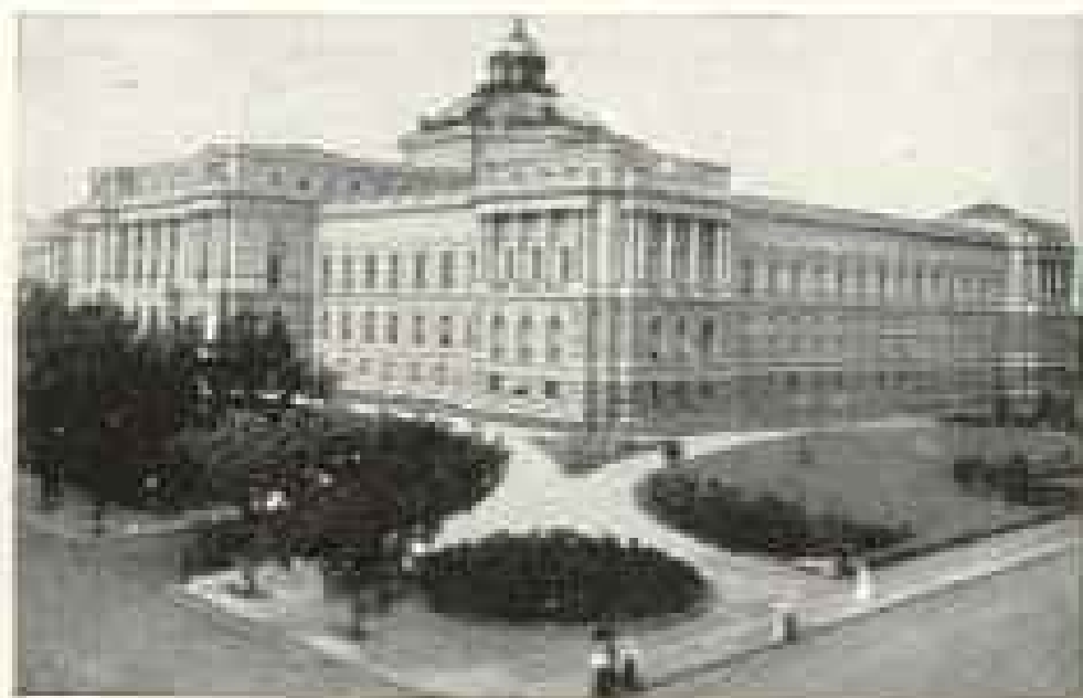
CONGRESSIONAL LIBRARY, WASHINGTON, D. C., EQUIPPED WITH MONARCH METAL WEATHER STRIPS. EQUIPPED BY THE JAMES B. HEN- DERSON CO., 303 DISTRICT NATIONAL BANK BUILDING, WASHINGTON, D. C.
