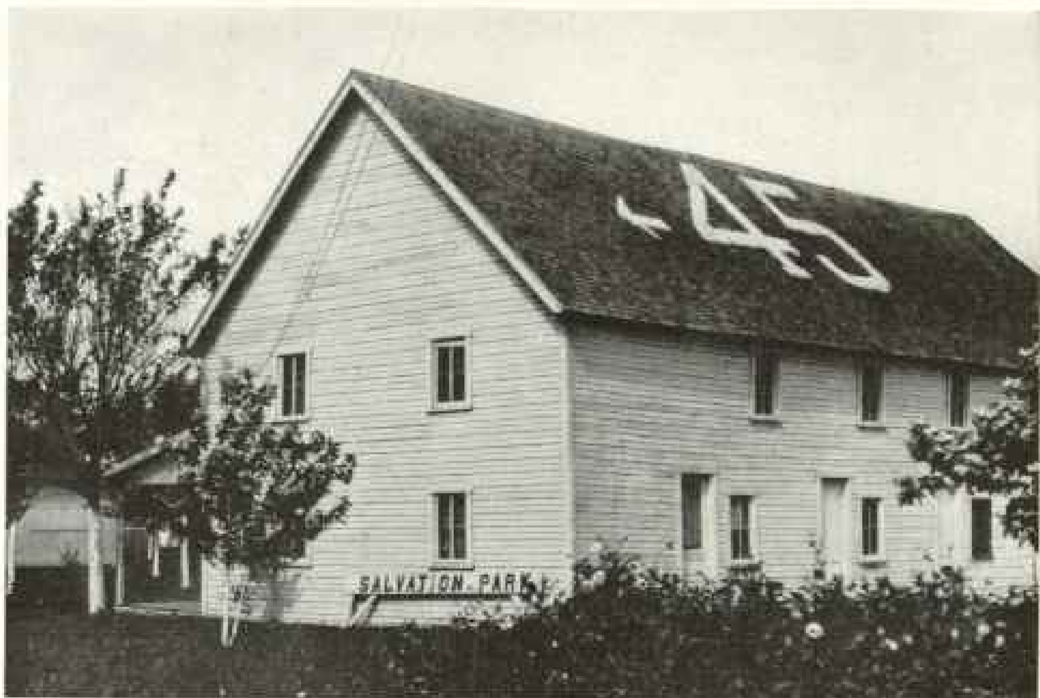
AN AVIATOR'S LANDING FIELD INDICATED BY HUGE NUMERALS PAINTED ON THE ROOF OF A BARN
