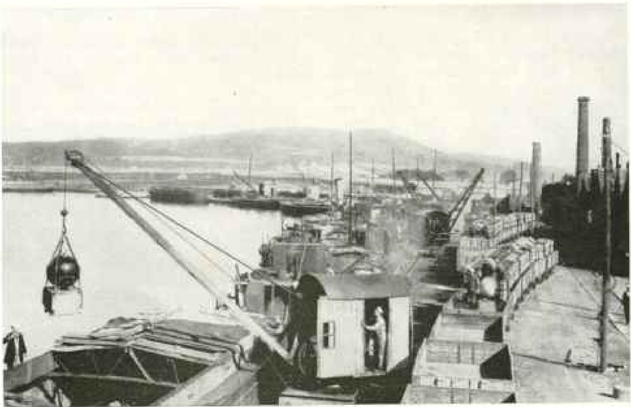
TRANSFERING MINES FROM RAILROAD CARS TO LIGHTERS A mine, shaped like a ball or an egg, is about one yard in diameter. With its iron box anchor, two feet square, and its wire mooring cable, it weighs 1,400 pounds.
