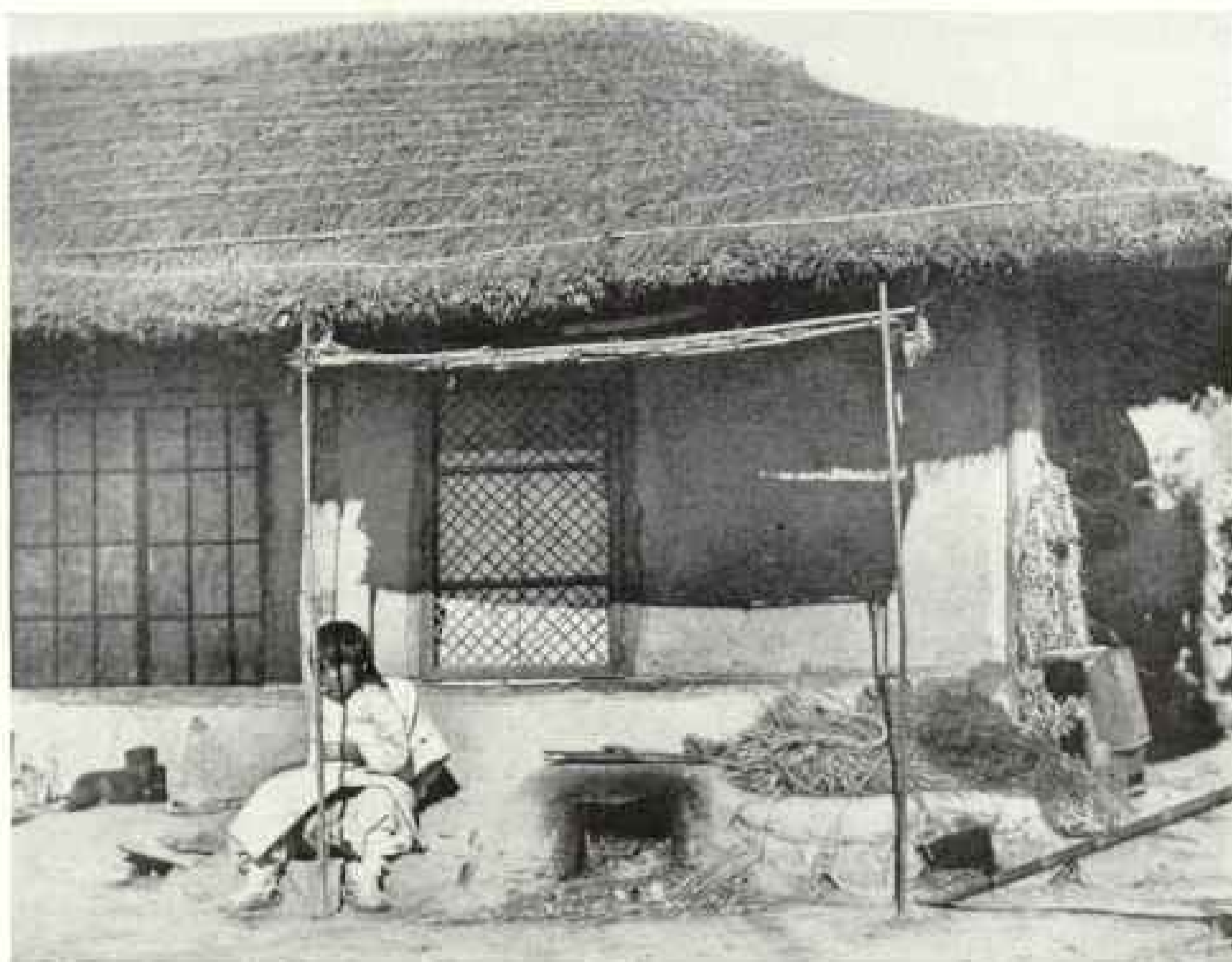
THE KOREANS HAD HOUSES HEATED BY HOT-AIR FURNACES LONG BEFORE WESTERN CIVILIZATION THOUGHT OF SUCH A CONVENIENCE.
