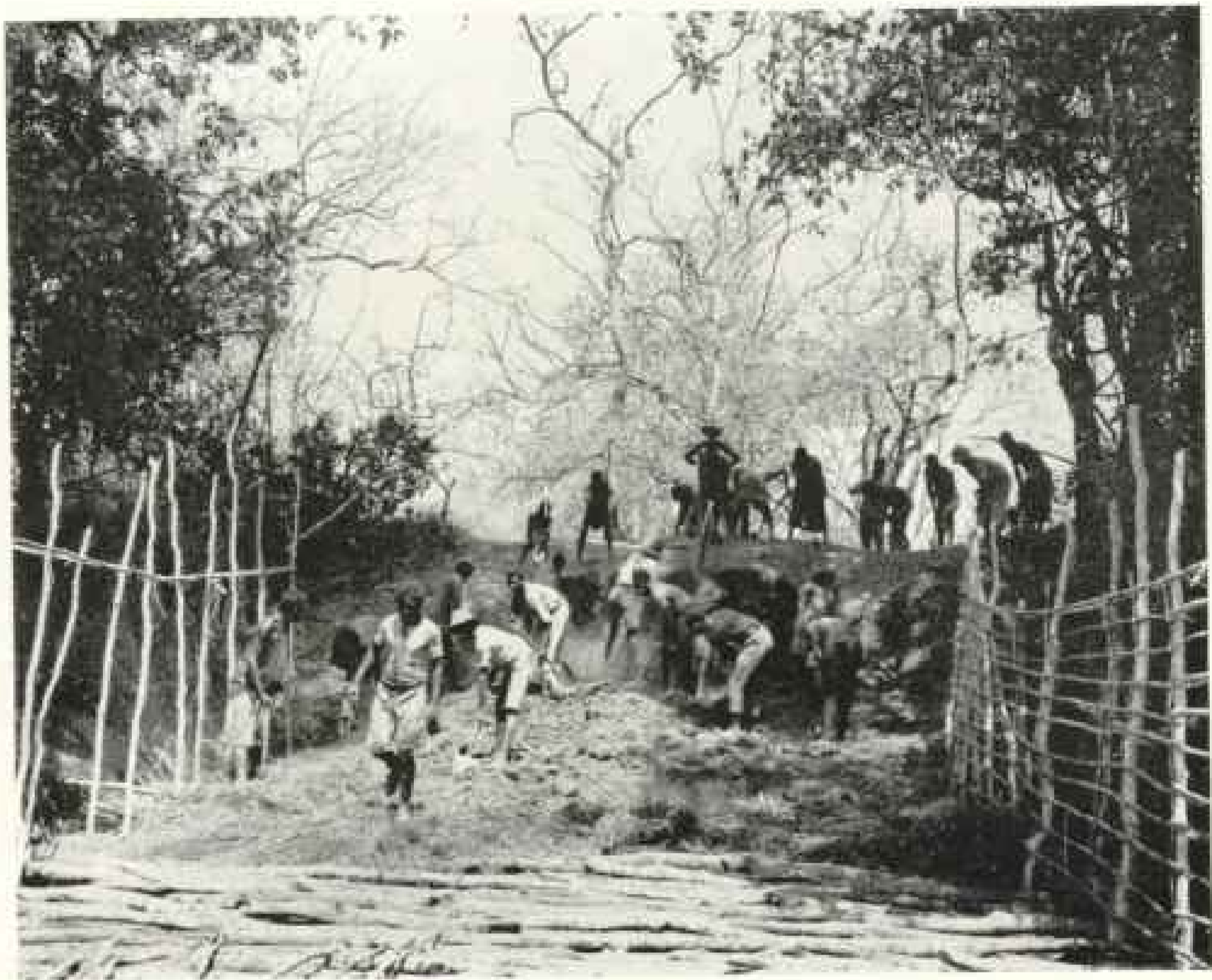
CARVING A PASSAGE THROUGH THE AFRICAN BUSH: BRIDGE-BUILDING
