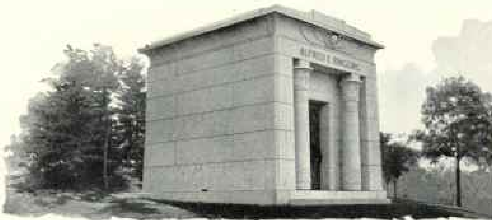
Alfred T. Ringling Mausoleum, Kenosha, N. Y. Egyptian Architecture, executed in Milford Pink Granite
