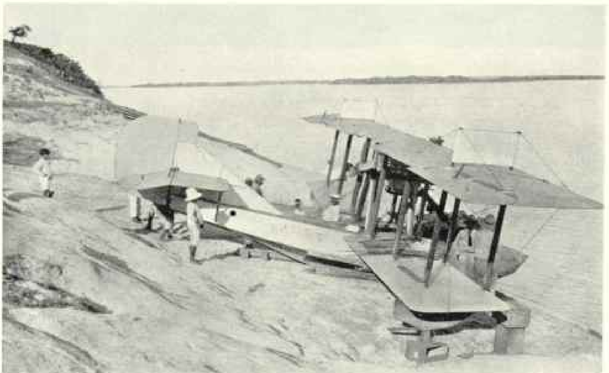
IN "DRY DOCK" AT BOA VISTA: REPAIRING THE HYDROPLANE HULL
