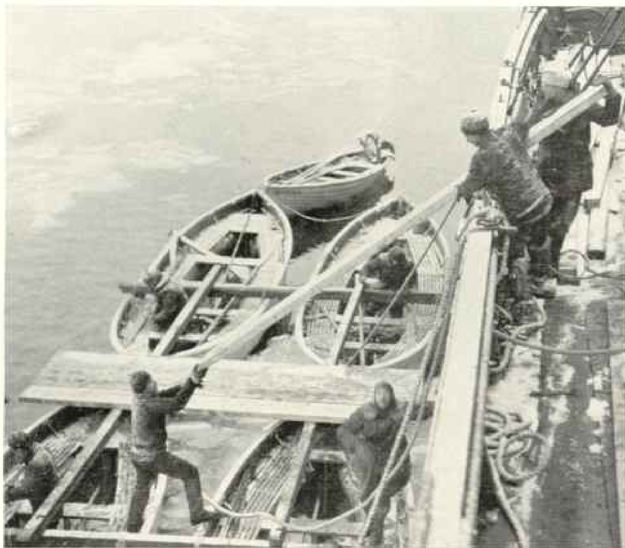
BUILDING THE PONTOON RAFT ON WHICH THE PLANE WAS TAKEN ASHORE
