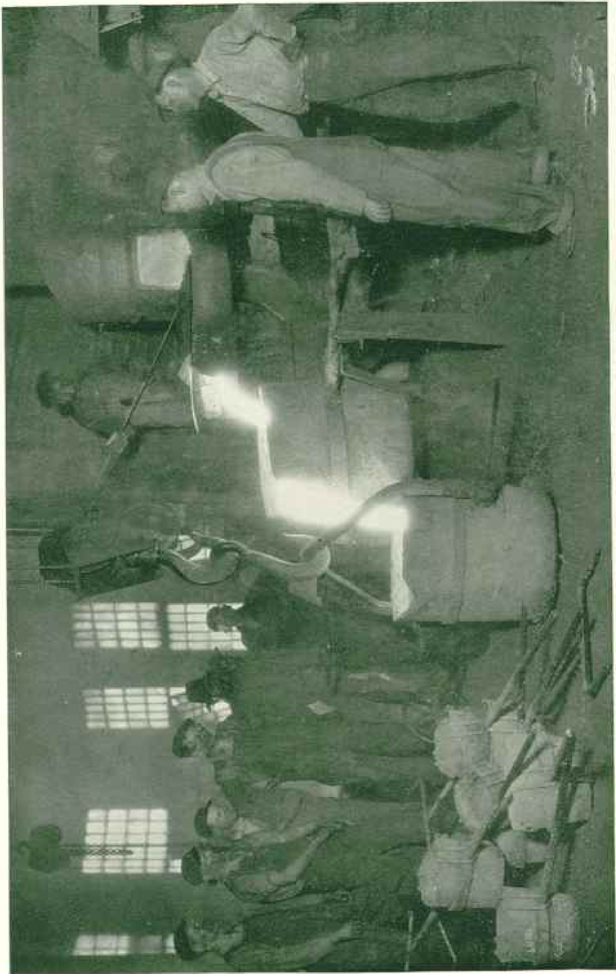
TAPPING A CUPOLA: INTERIOR OF AN IRON FOUNDRY IN MACON
