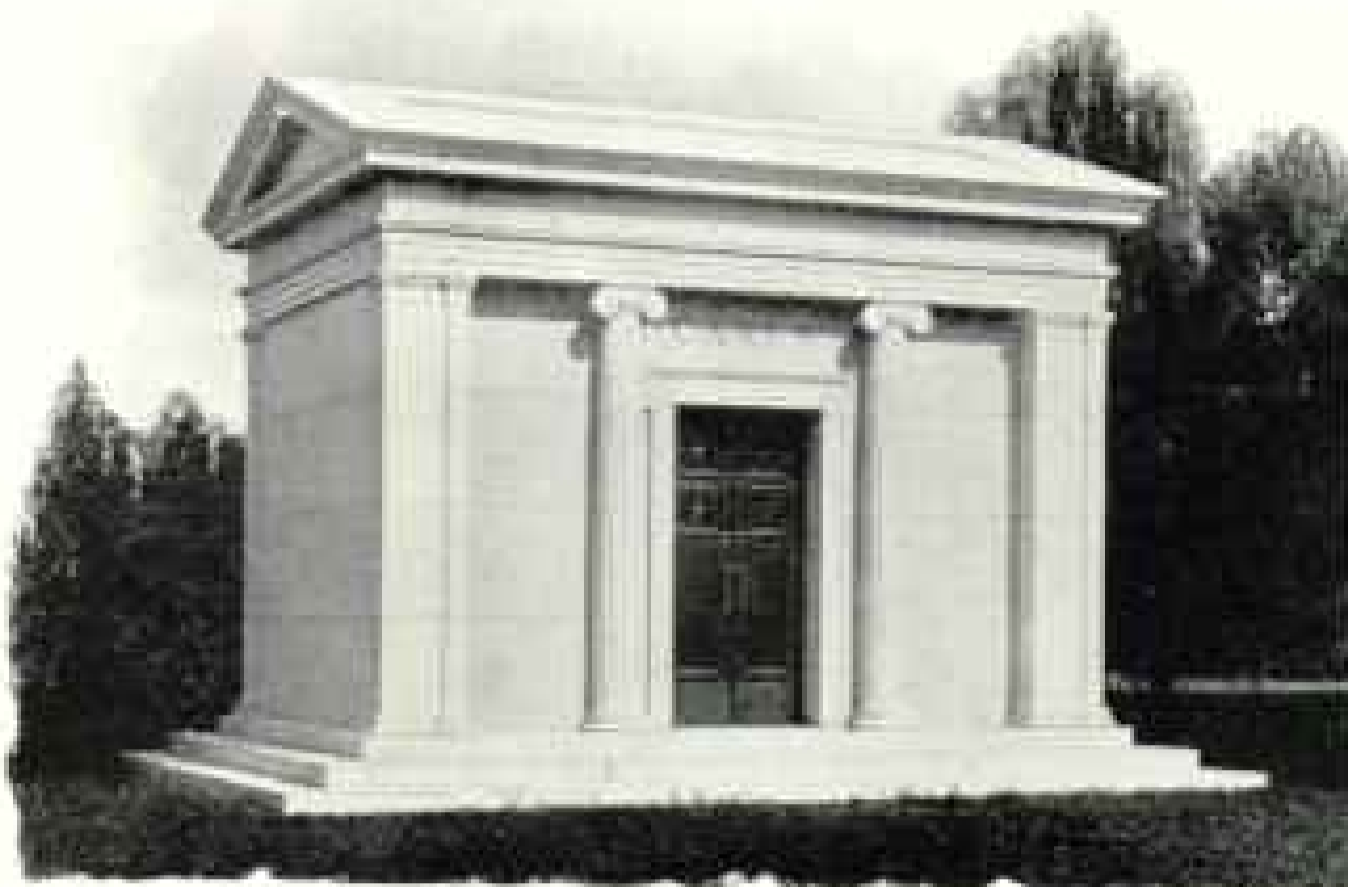
The Carew Mausoleum is erected in Spring Grove Cemetery, Cincinnati, Ohio. Victoria White Granite was used in the construction.
