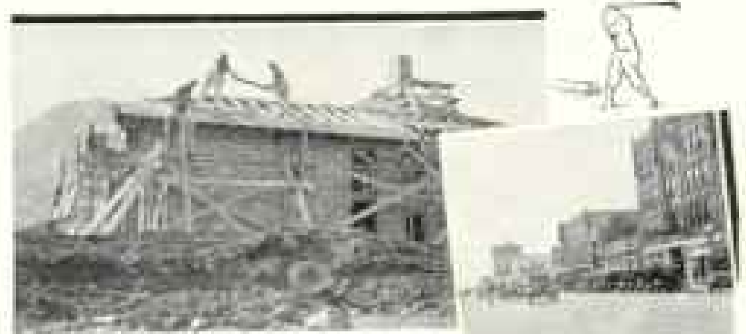
Building Under Way—Jan-28-1920 Right—Imperial—Feb 2-1927
