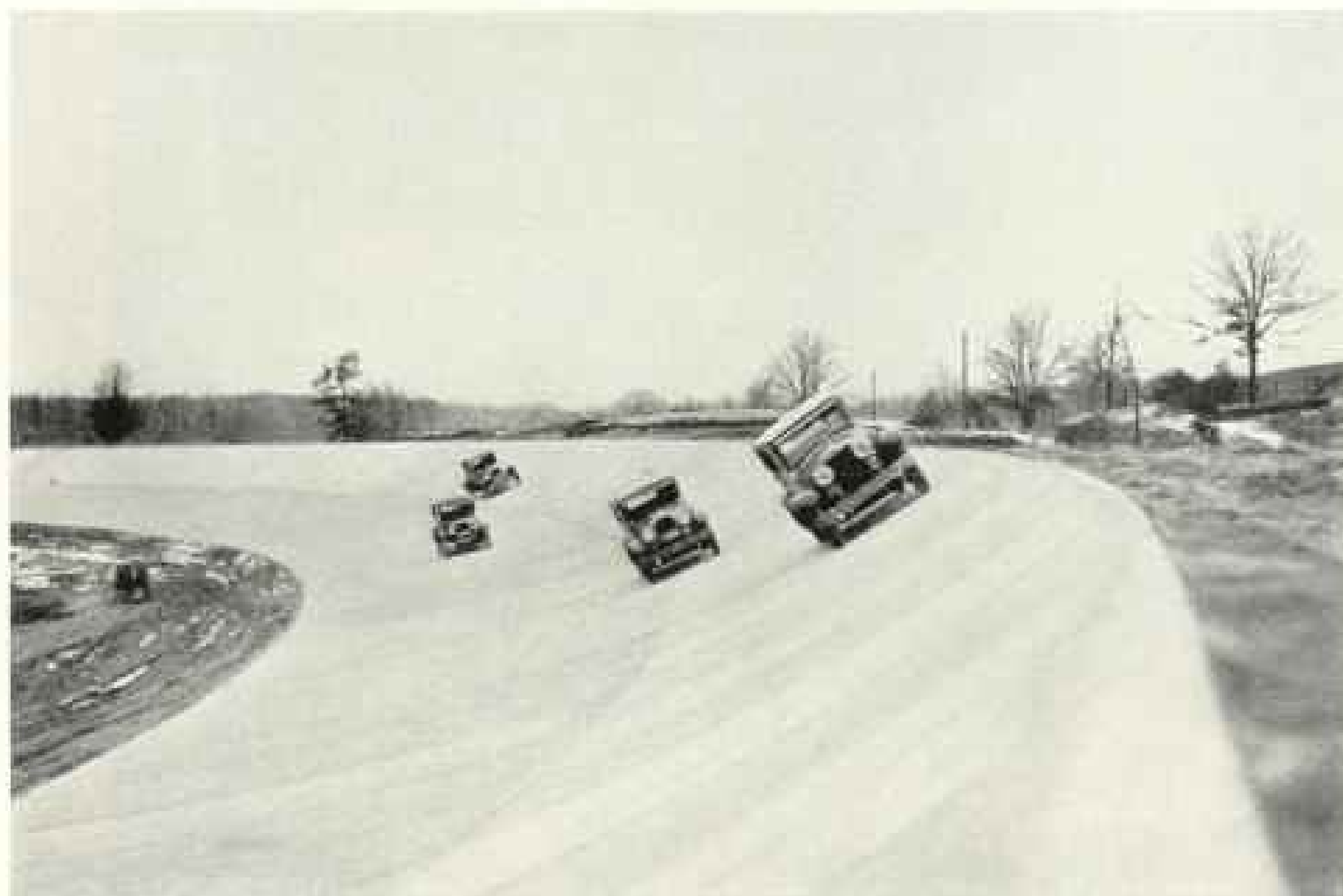
Photograph from General Motors
