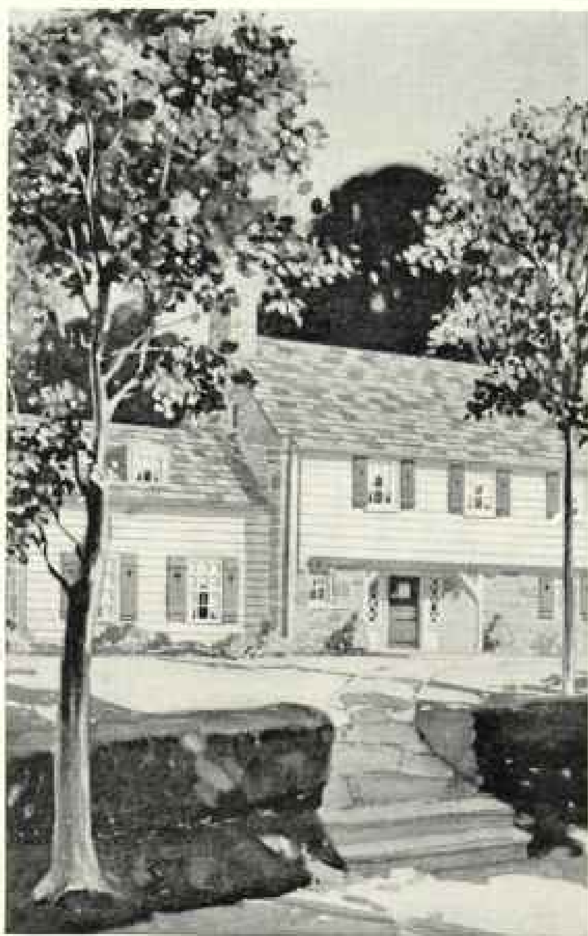
Johns-Manville Asbestos Shingles on the Residence of Dr. H. E. Robinson, Pleasantville, N. Y. Architect—James R. Thompson
