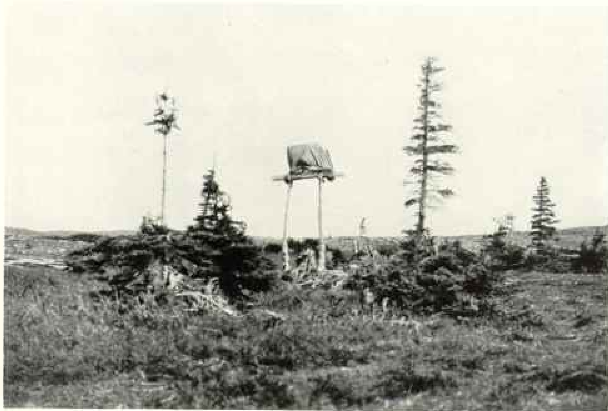
PROVISION CACHES REST ON STRIPPED POLES
