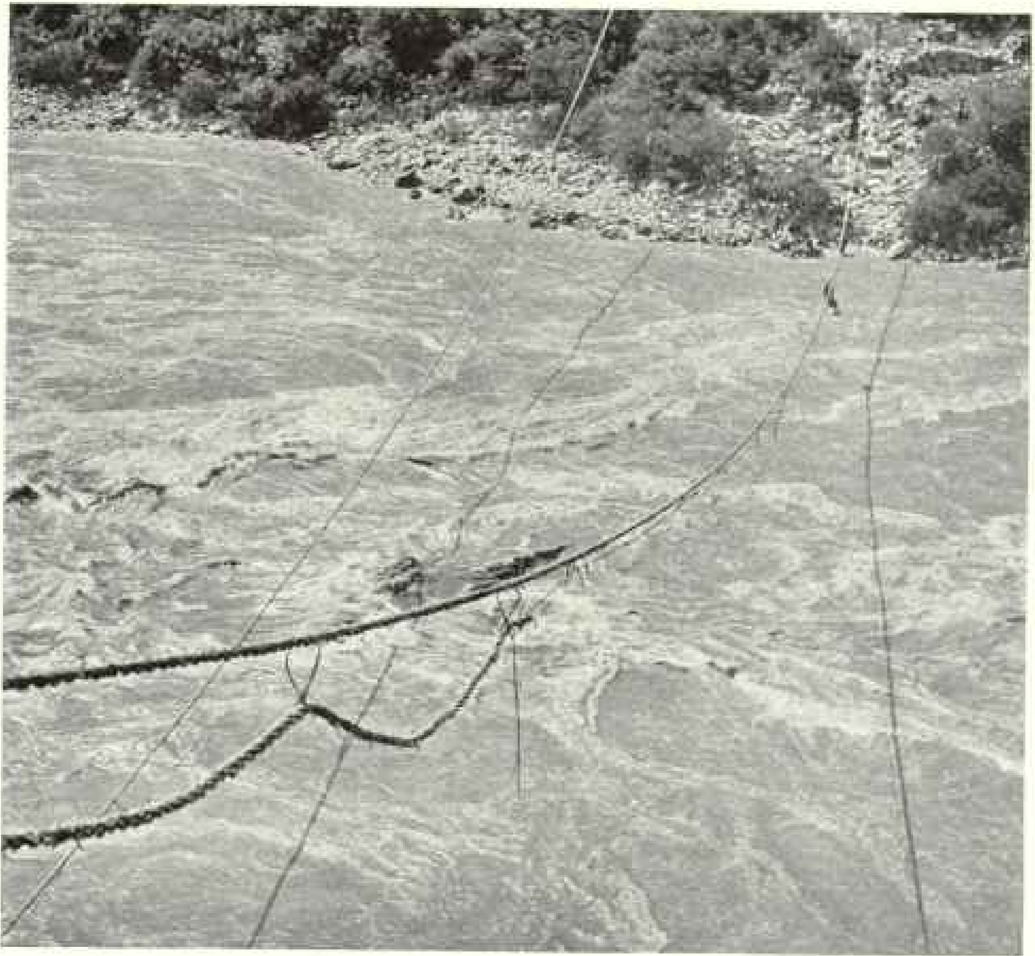
SUSPENDING A NEW BRIDGE ACROSS THE YALUNG
