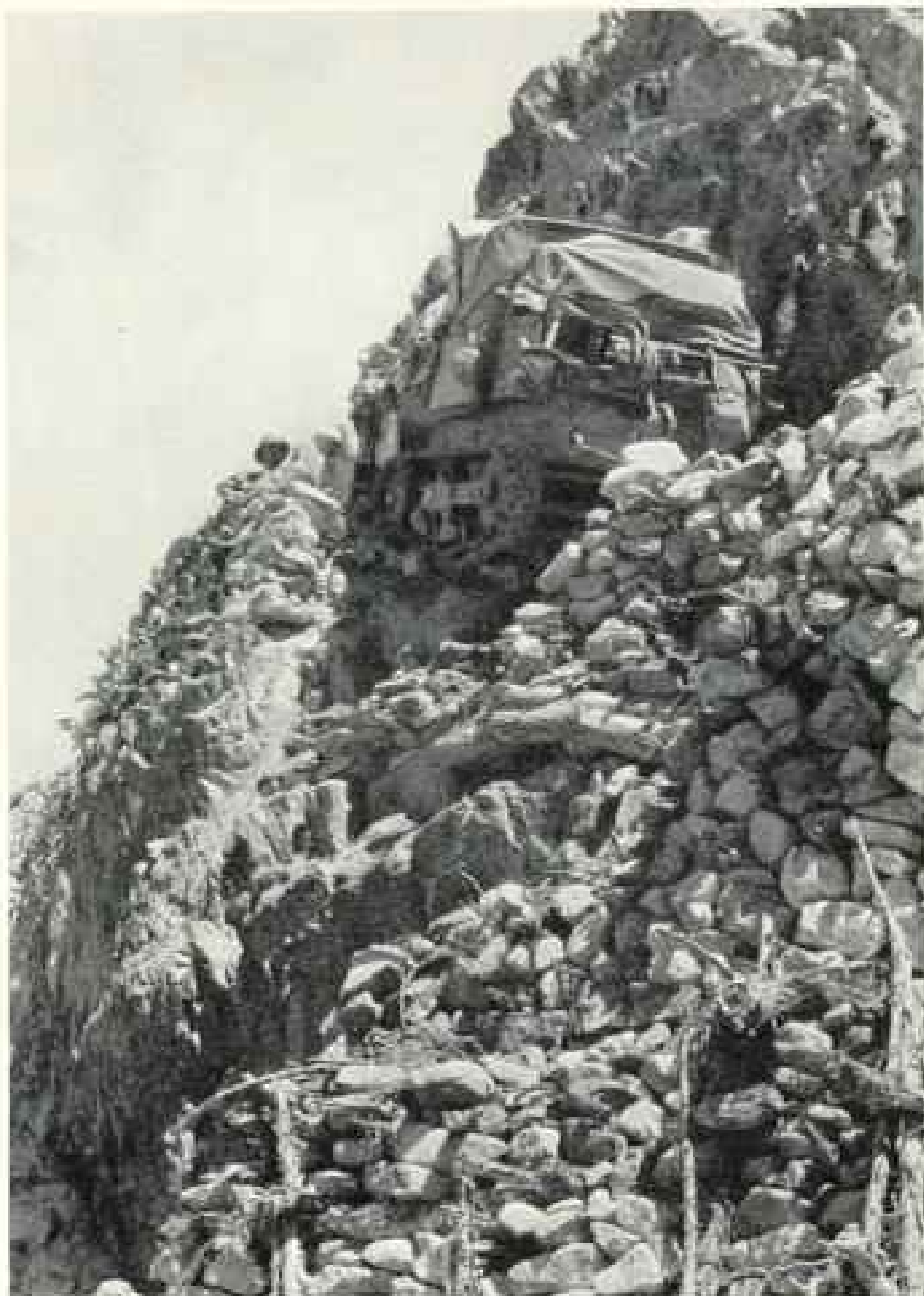
ONLY A FEW LOOSE STONES BETWEEN LIFE AND DESTRUCTION
