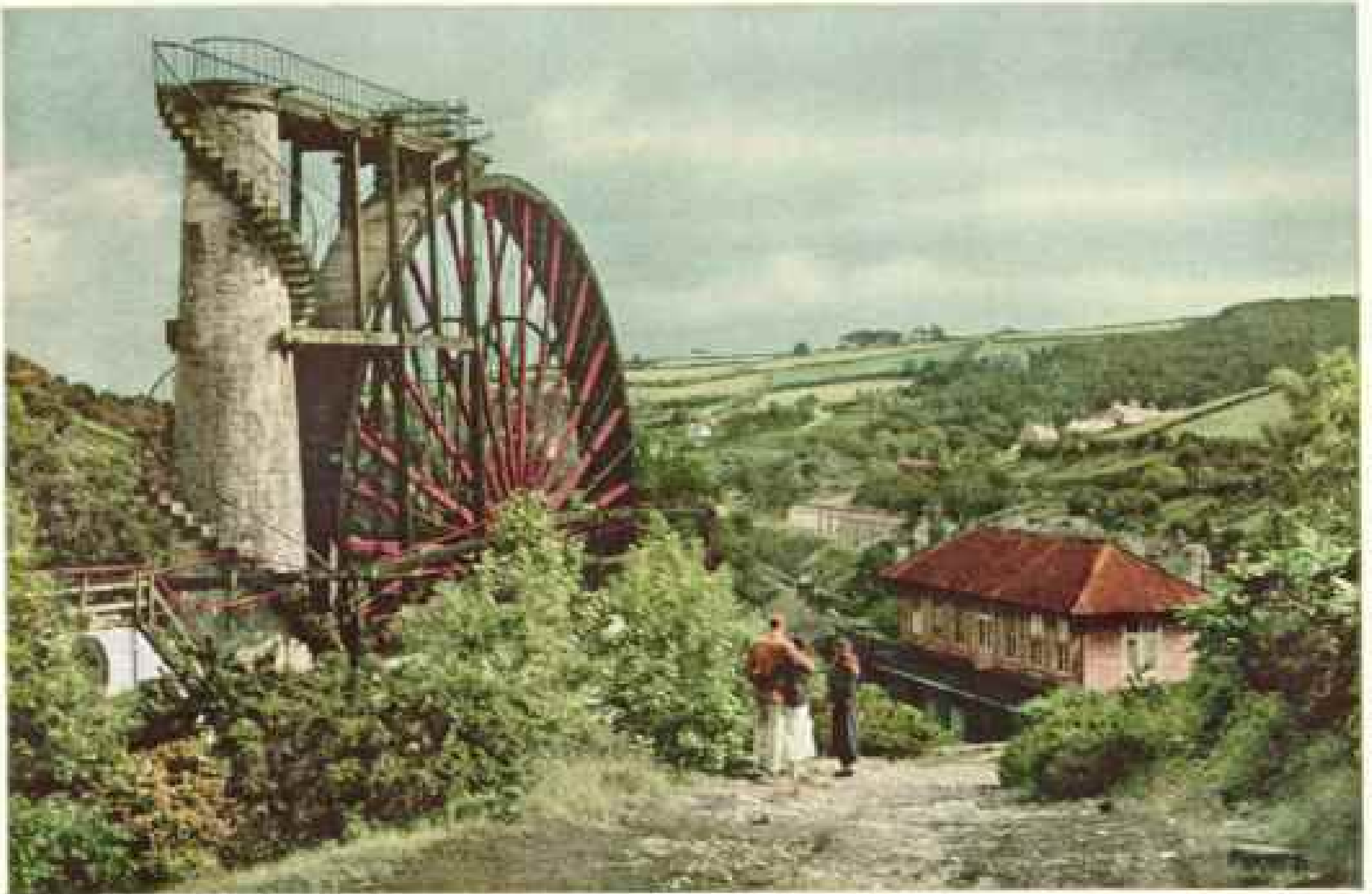
"LADY ISABELLA" WAS BUILT TO PUMP WATER FROM LANEY LEAD MINES. Named for the wife of a Manx governor, the big wheel, now idle, was turned by water piped down from the hills. Near-by mines were once among Britain's most productive.
