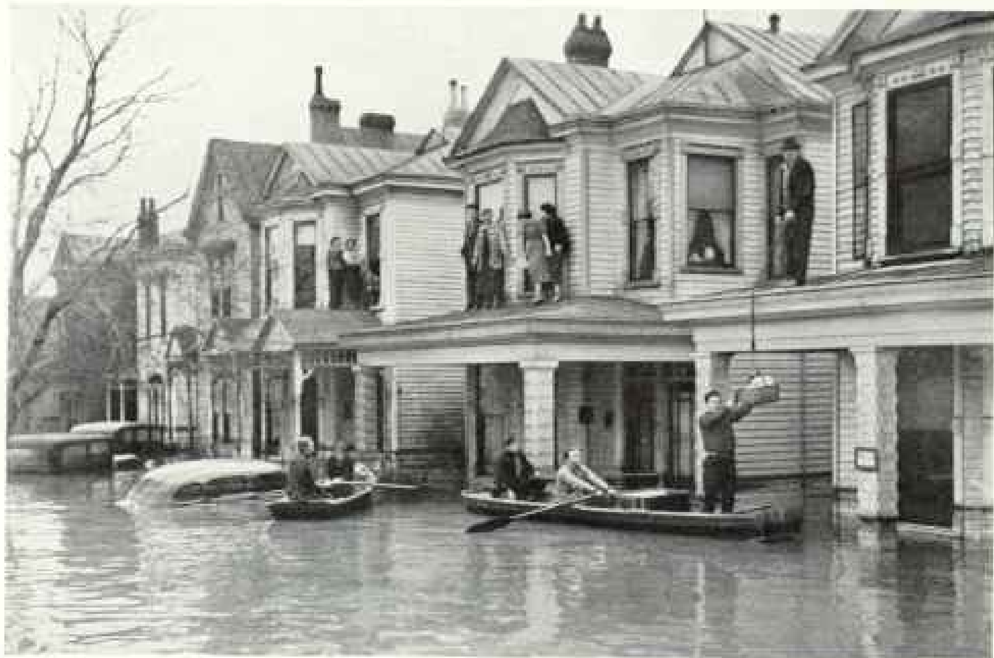
Photograph from Acme
