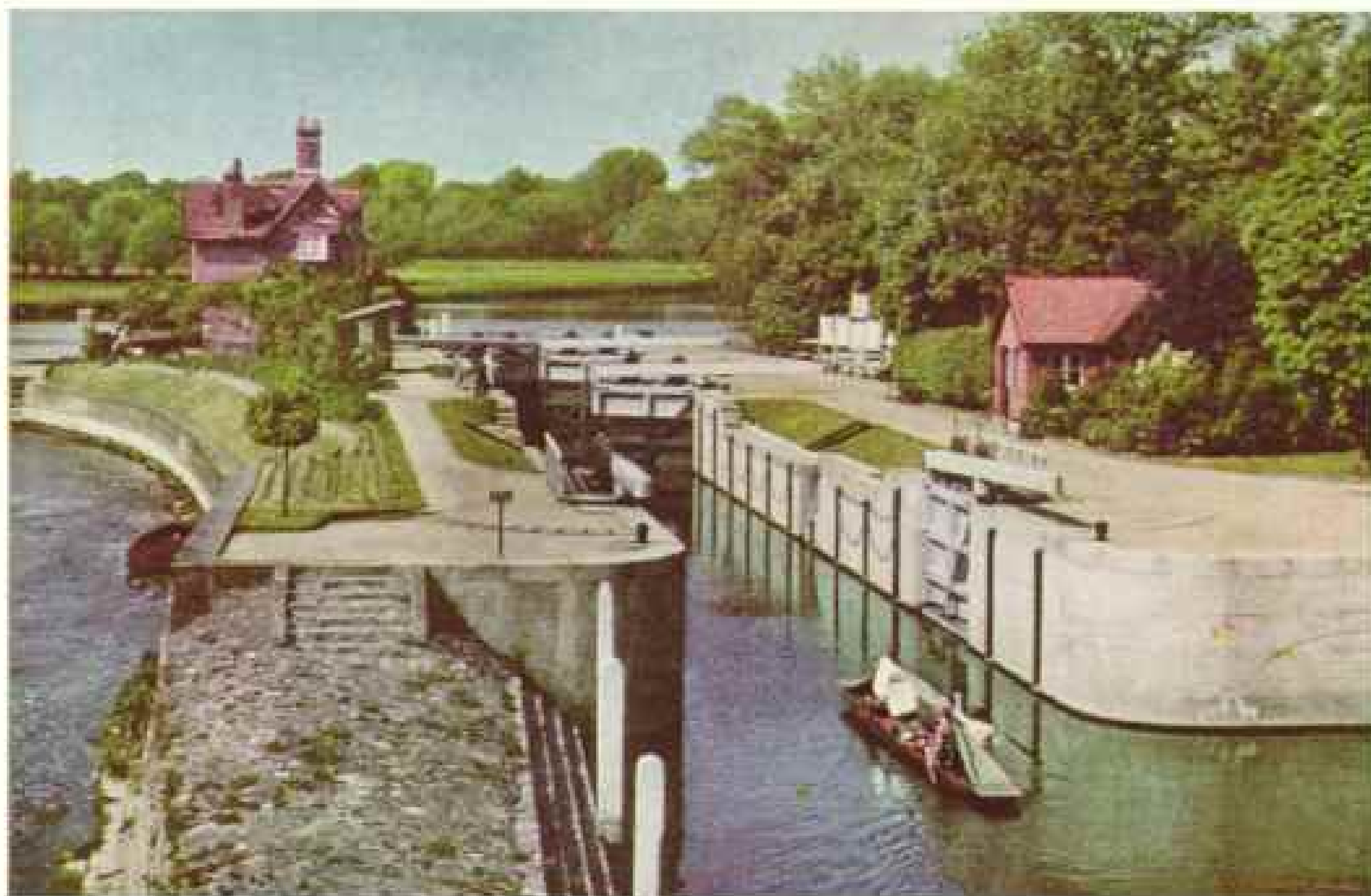
AMPLE BOATING WATER IS HELD IN UPPER THAMES BY 49 LOCKS AND DAMS. Were such barriers as this at Goring swept away, the river, from Oxford down to London's outskirts, would fall so fast that boat traffic would be difficult.
