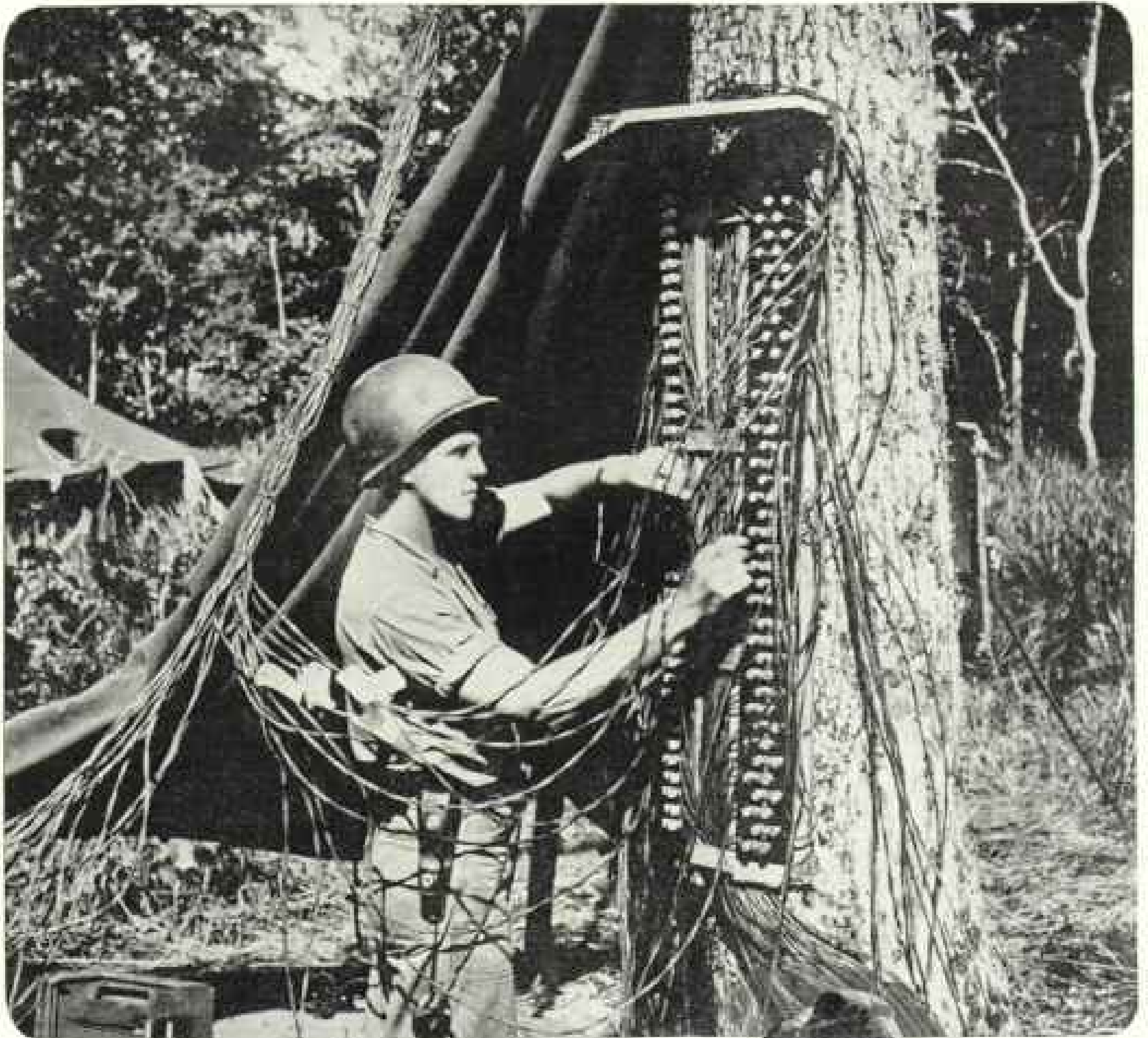
U. S. Marine setting up a telephone switchboard on an island "somewhere in the Pacific"
