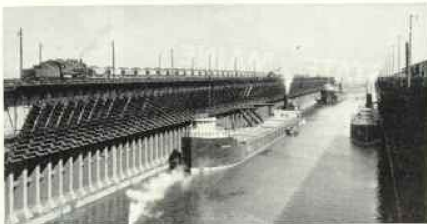
Allouez docks rise 80 feet above water. During the 1944 ore season a total of 2,184 Great Lakes boats were loaded here.
