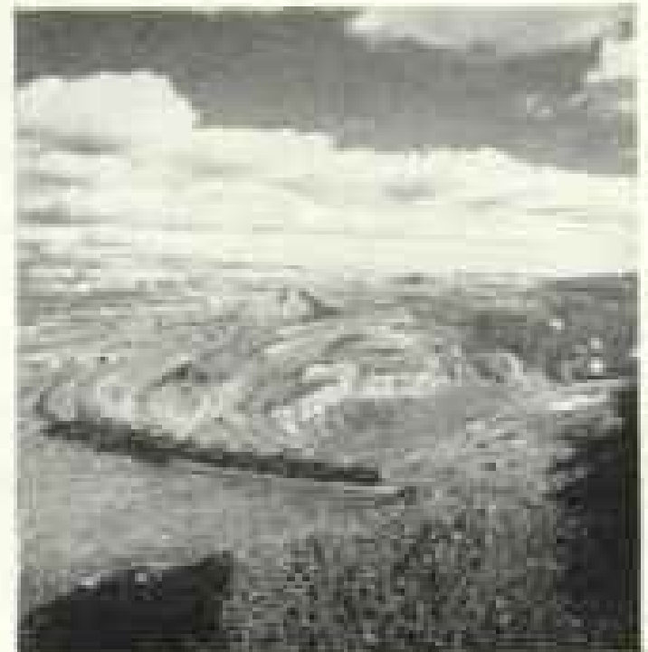
World's largest open pit mine is on the Minnesota iron range. The pit is nearly 4 miles long, over a mile wide and 600 feet deep.
