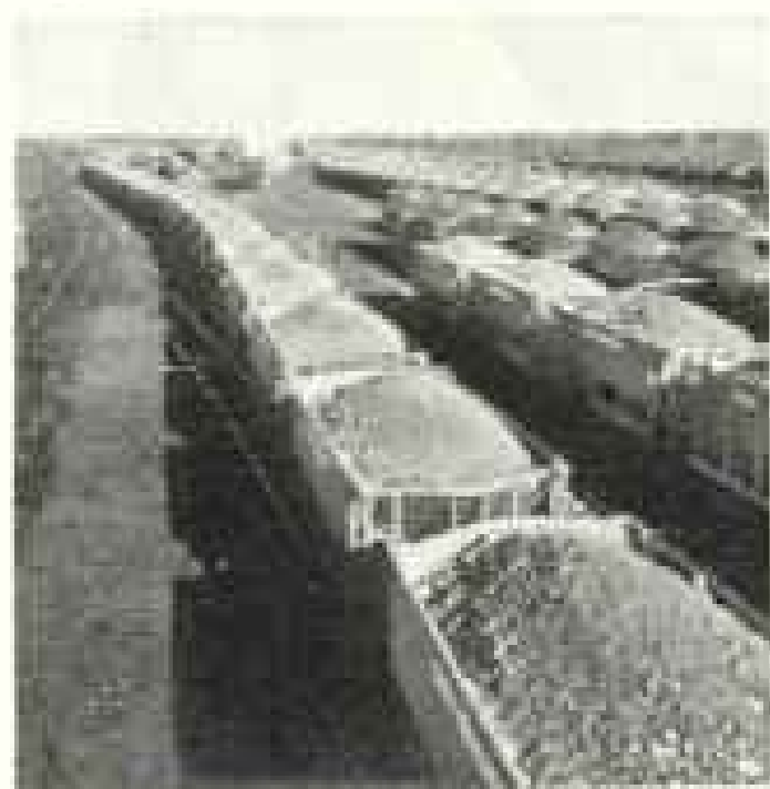
A section of G.N.'s classification yards where ore trains deliver cars for weighing and sorting.
