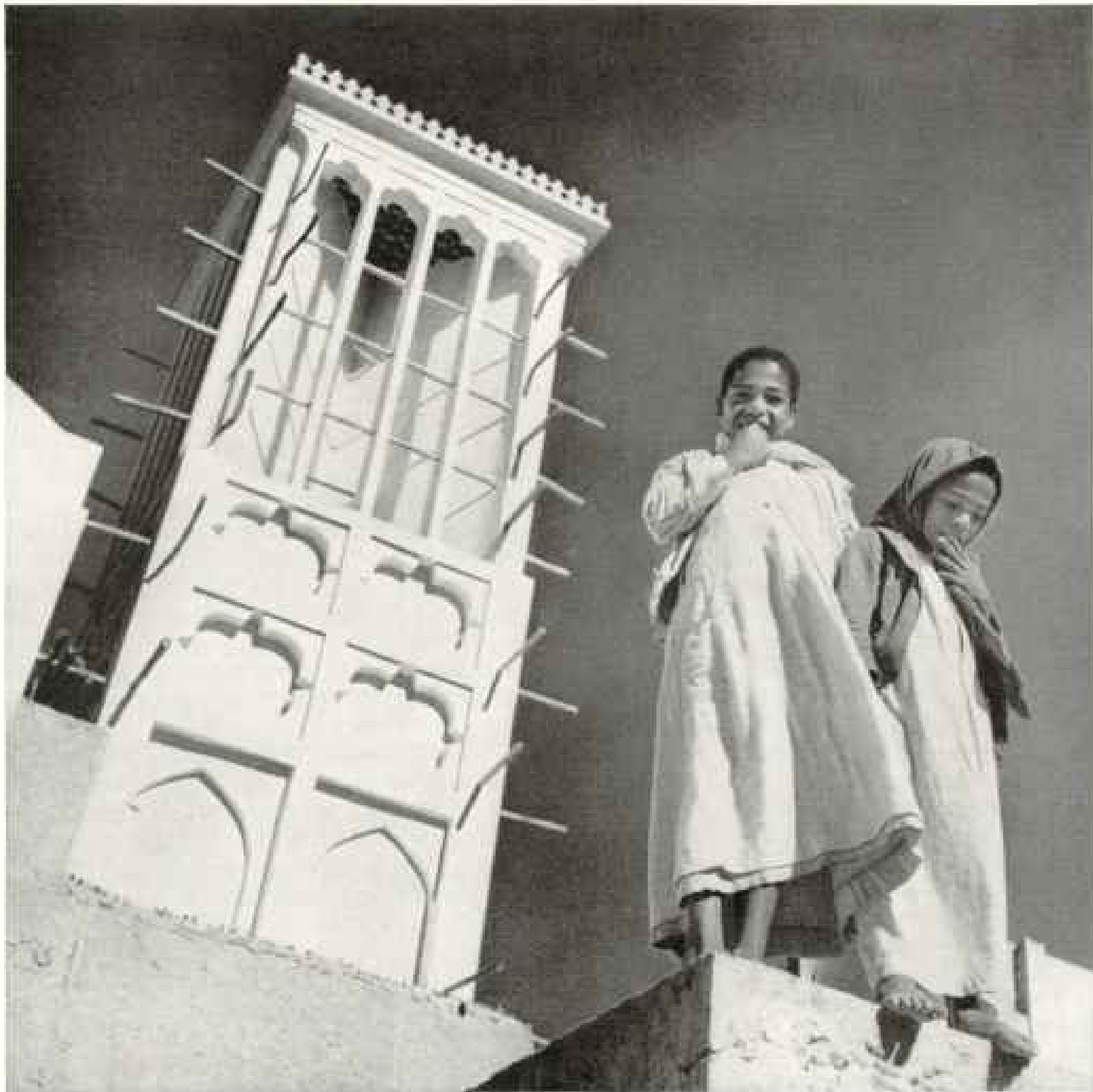
Marco Polo, Centuries Ago, Saw Such Air-conditioning Towers Beside the Persian Gulf. Catching any possible breeze in one of its four triangular shafts, this ventilator near the American Mission Hospital serves as a wind scoop, pouring cool air into the home (page 209).
