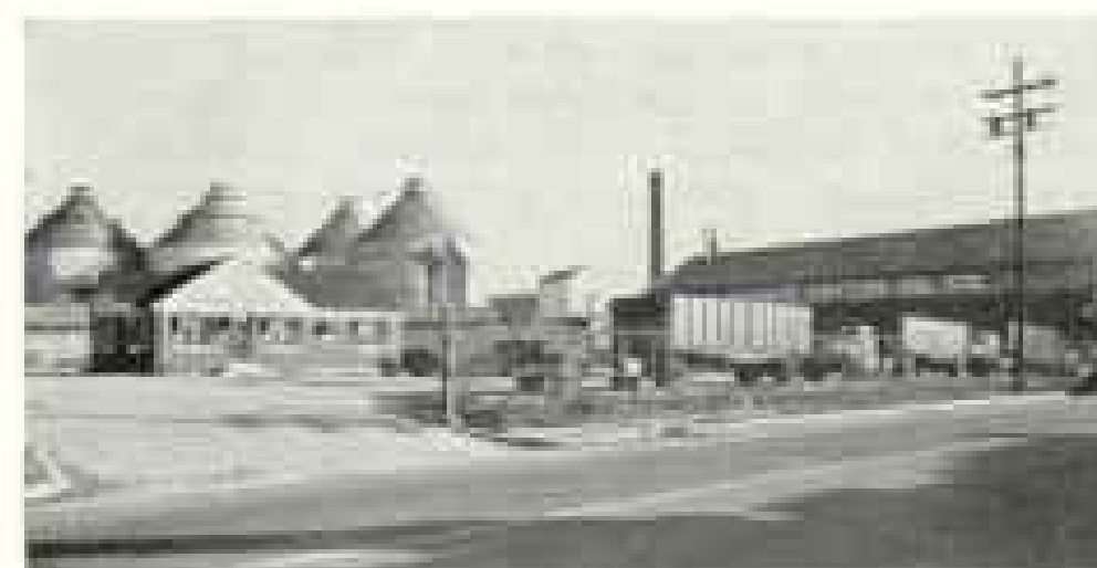
IN MISSISSIPPI —THE BUCKEYE COTTON OIL COMPANY, Jackson. Cottonseed from Mississippi's famed cotton fields are the raw materials used by this plant to manufacture high quality vegetable oil for shortening and salad oil, high protein livestock feeds, cotton linters and cellulose.
