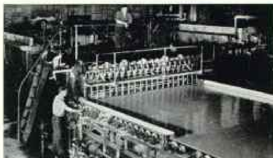
Part of the Machine on Which Pulp Fibers Are Formed into a Web of Paper
