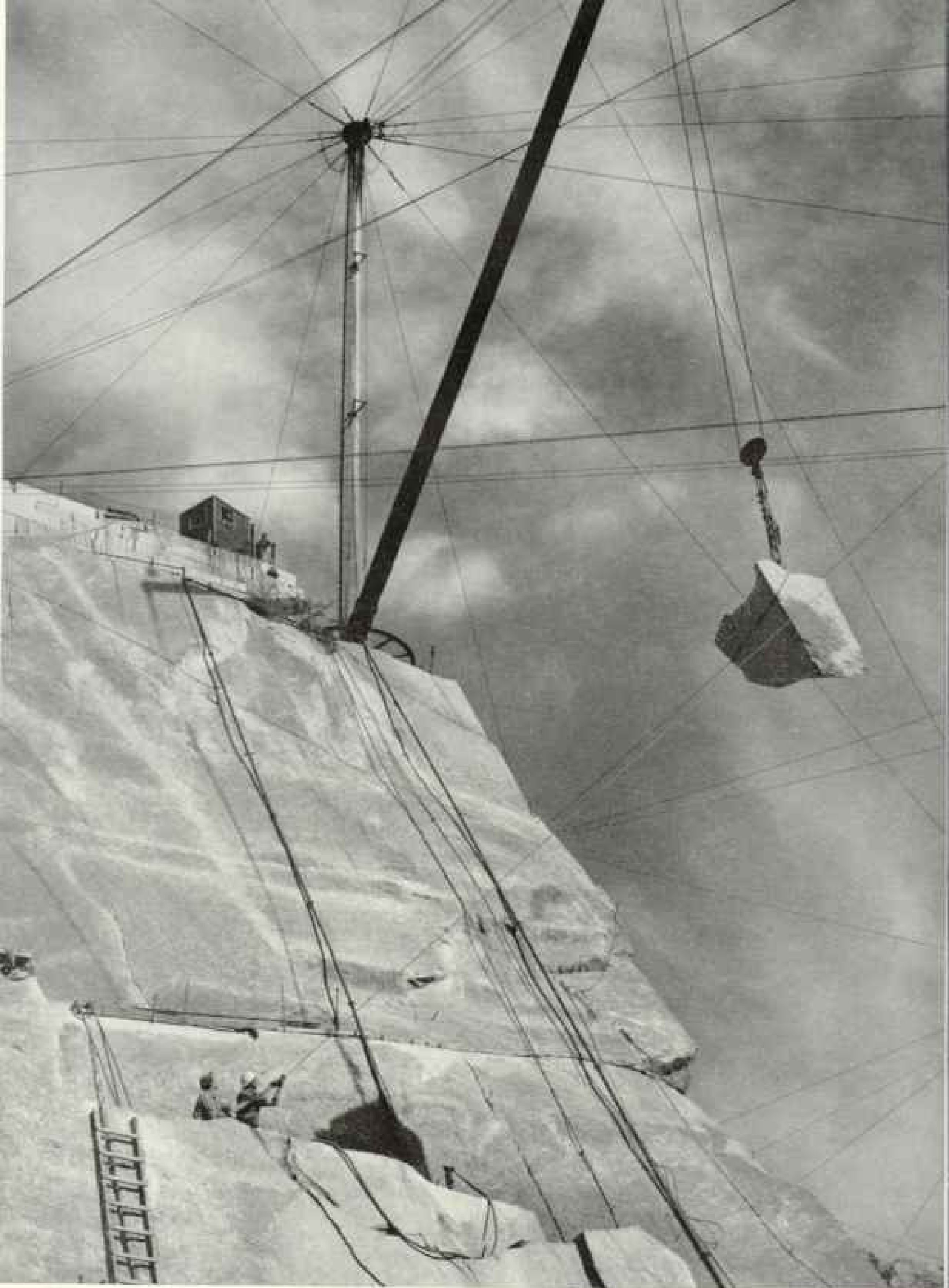
25 Tons of Granite Dramatically Rise from the 300-foot Depths of Rock of Ages Quarry This 40-acre pit is near Barre, Vermont, "Granite Center of the World." Derricks, beneath an umbrella of cables, are Oregon firs, 115 feet long and 3 feet thick. Pipes carry compressed air to drill crews (opposite page).
