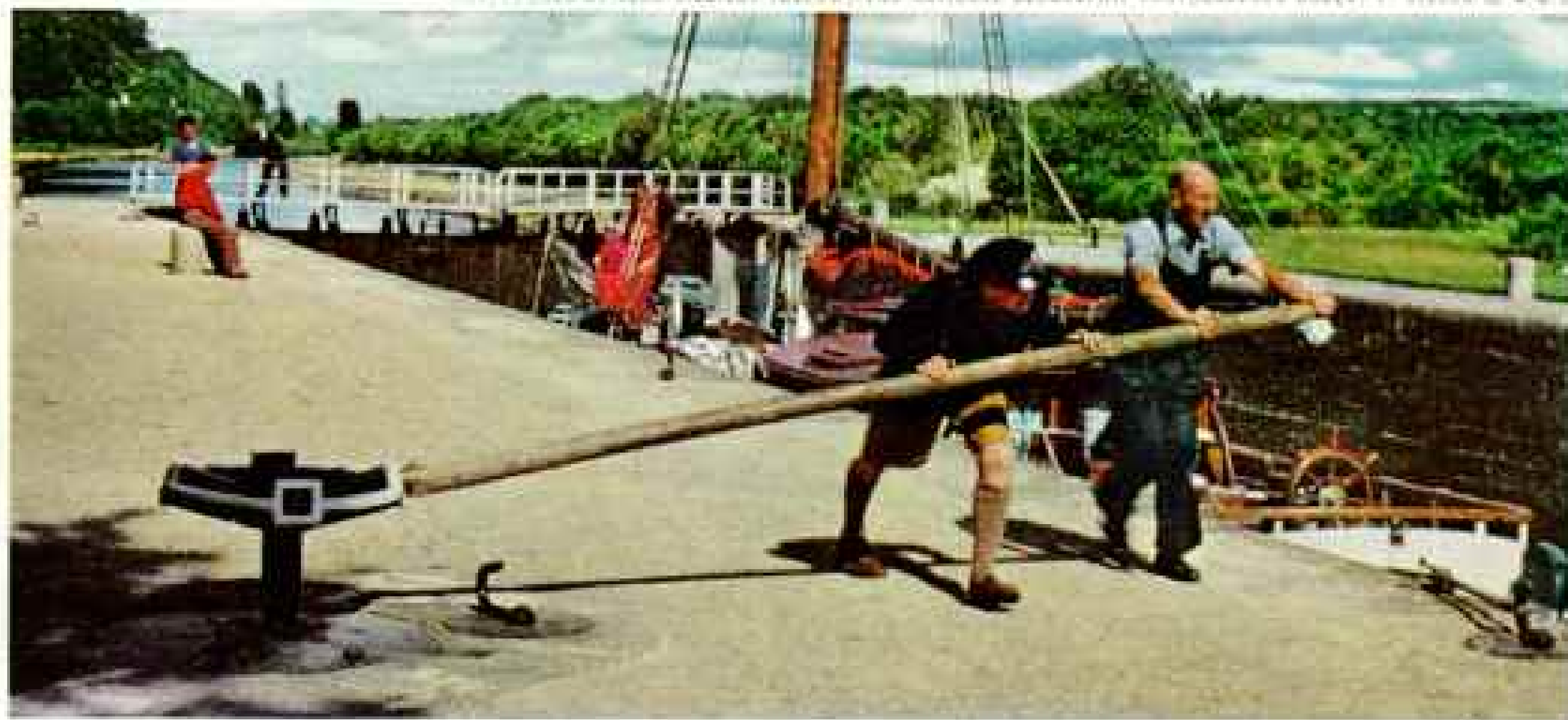
Heaves on a capstan bar swing lock gates on Scotland's Caledonian Canal. Cristoden's crew often helped keepers walk the gates open or shut.
