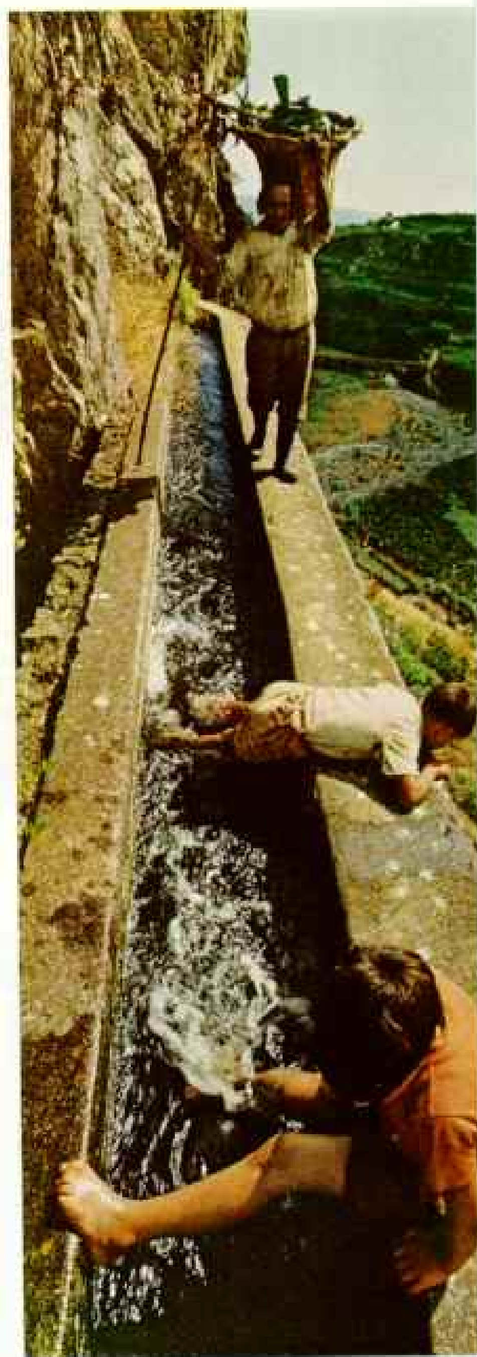
Watercourse and walkway, a levada (above) affords a footpath to and from emerald uplands. A surefooted farmer carries bananas on his way to market. Tapping streams in the island's precipitous spine (facing page), levadas provide water for irrigation and electric power.
