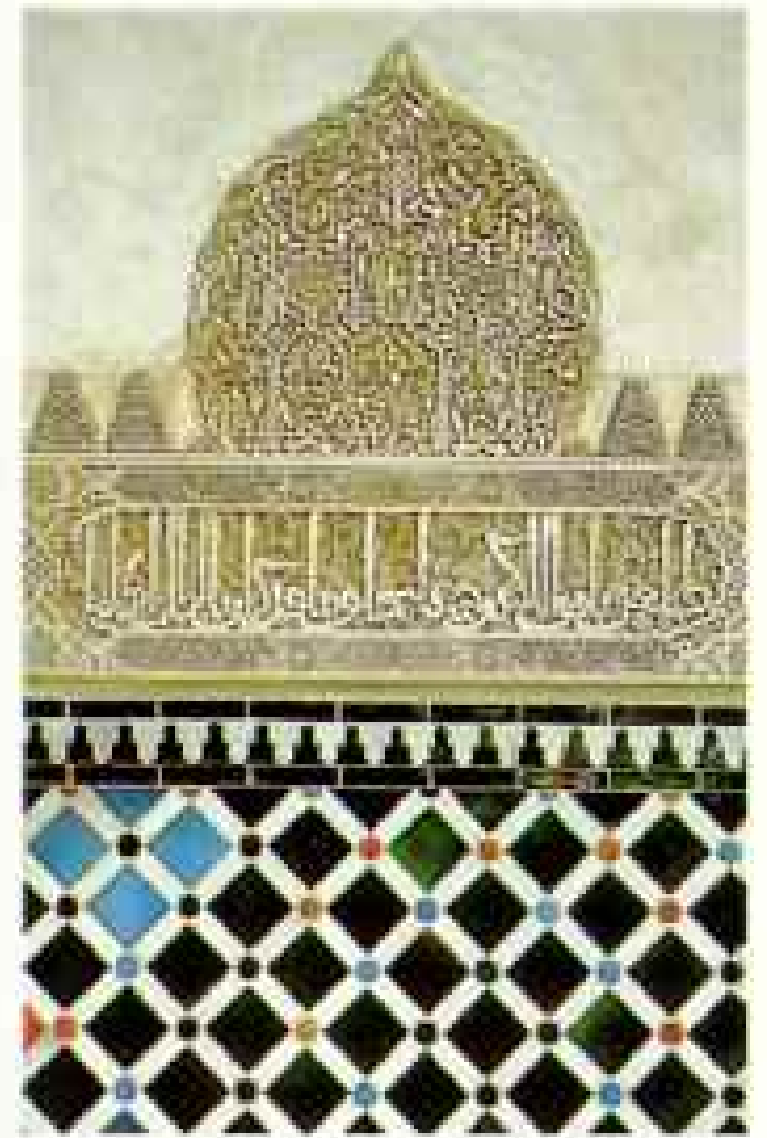
ARTFUL ARABESQUES and vivid tile work adorn the Alhambra in Spain (above) and the king's palace in Fez, Morocco (facing page). The technique of carving plaster walls with intricate, geometric patterns was widely used by Moorish architects and is still practiced today by craftsmen restoring buildings in Toledo and Granada.
