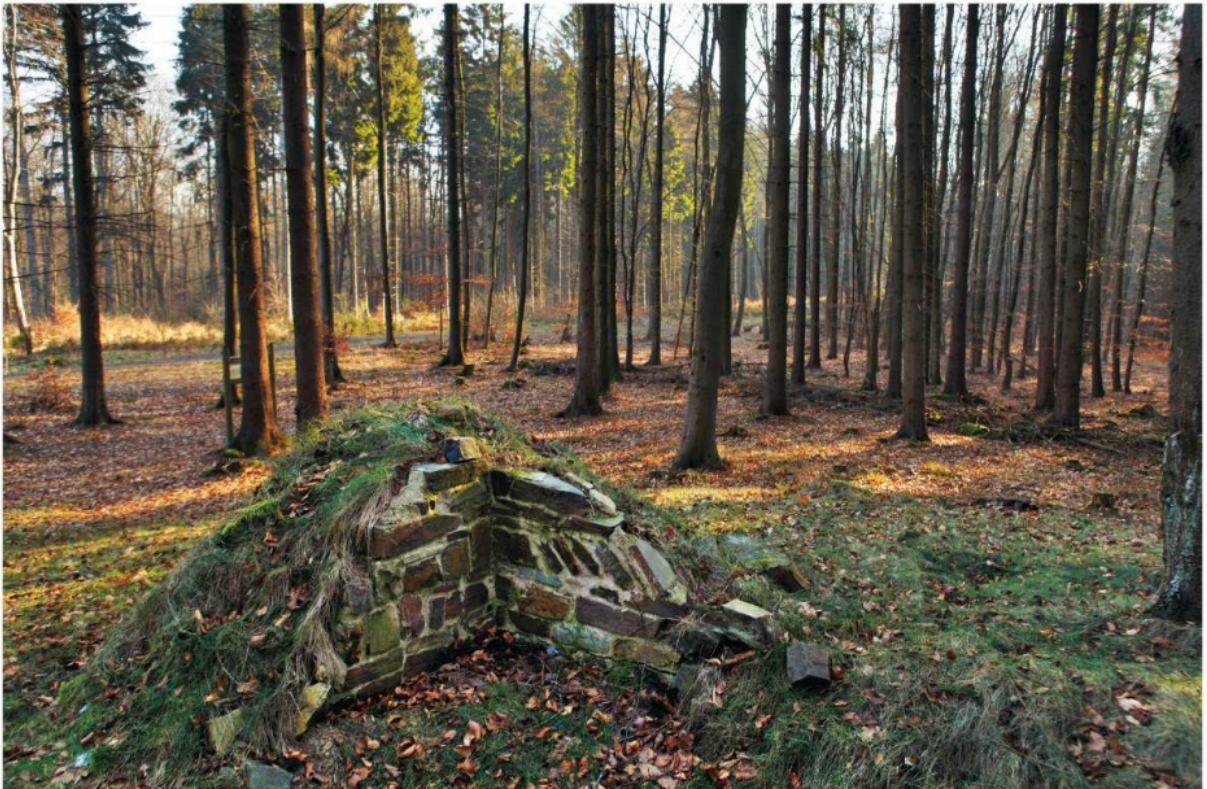
BECHELN, GERMANY Only a few stone foundations remain from the more than 800 watchtowers built by Roman soldiers along 342 miles of the frontier linking the Rhine and Danube Rivers.
