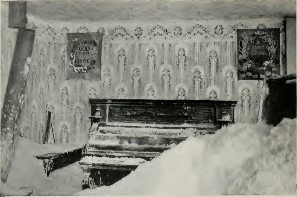
A HOUSE AT KODIAK RUINED BY AN AVALANCHE OF ASHES FROM A HILLSIDE
