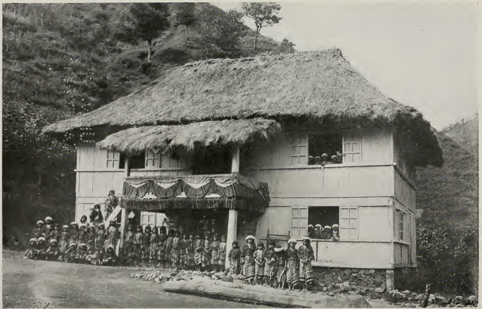
A SCHOOL-HOUSE BUILT BY BENGUET IGOROTS AT KABAYAN
