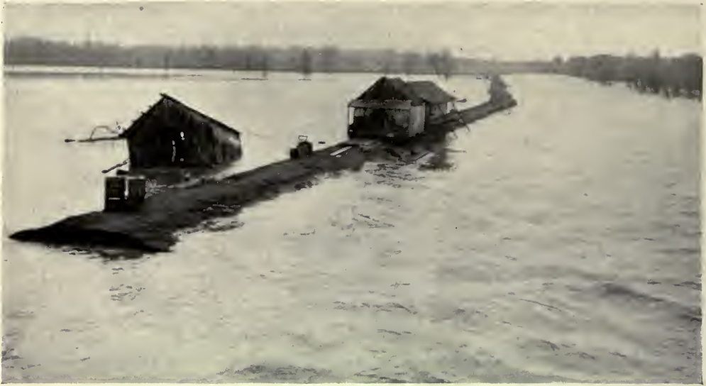
A BROKEN MISSISSIPPI RIVER LEVEE AT LUCCA, ARKANSAS
