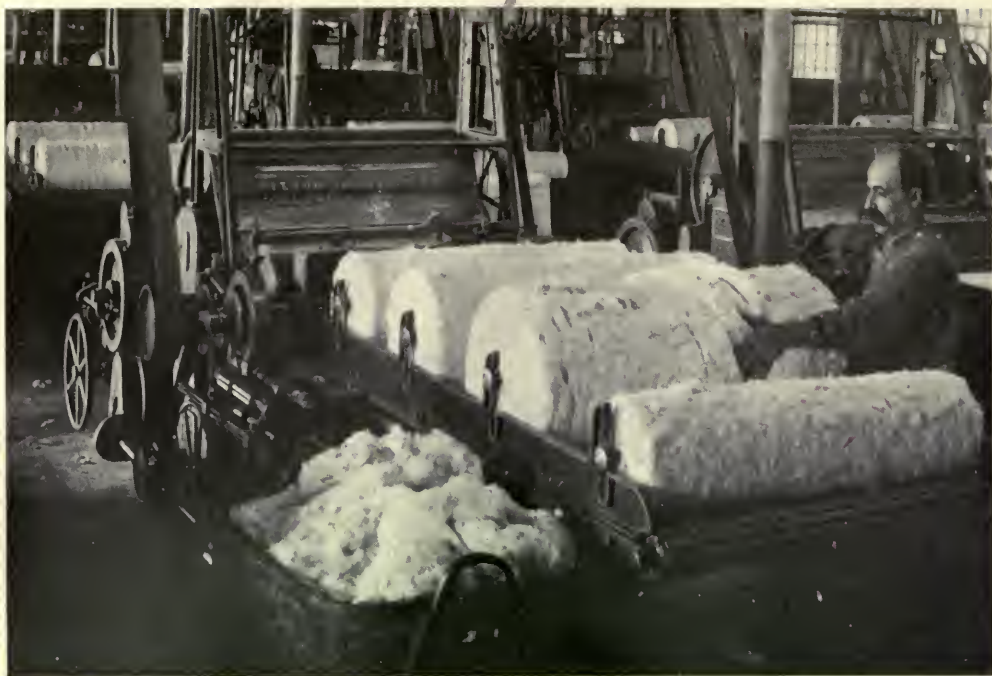
THE INTERMEDIATE PICKER, WHICH CONTINUES THE WORK OF CLEANING RAW COTTON
