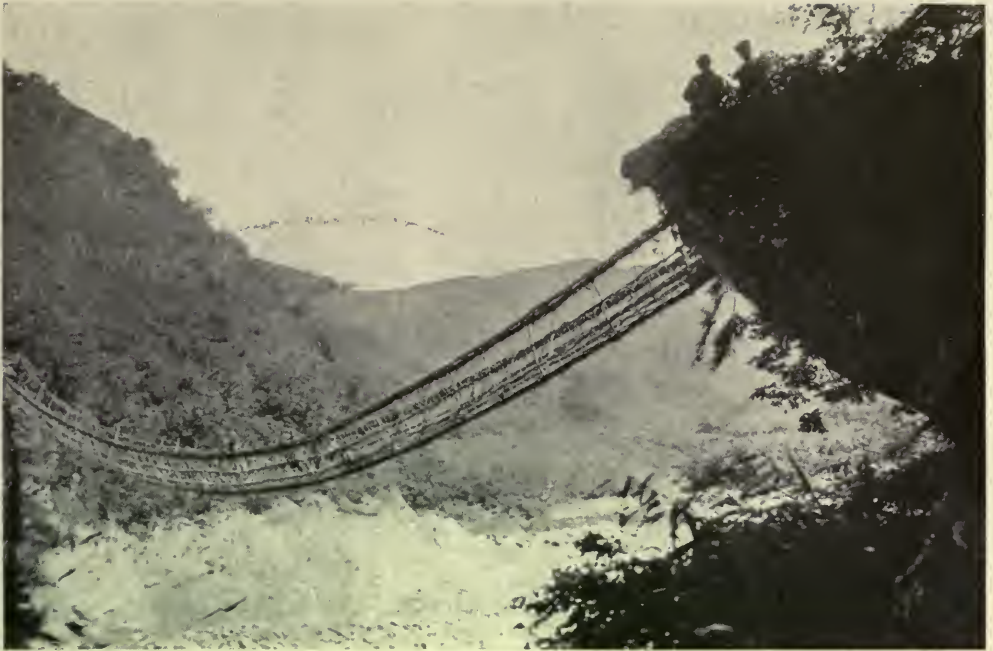
A RATTAN SUSPENSION BRIDGE CONSTRUCTED BY THE JAPANESE IN THE SAVAGE COUNTRY
