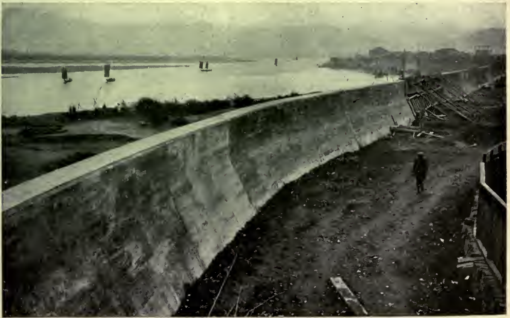
VIEW OF THE DAITOTEI BUND SHOWING THE TYPHOON WALL: TAKEN FROM THE EXTREME SOUTHERN END OF TAIHOKU
