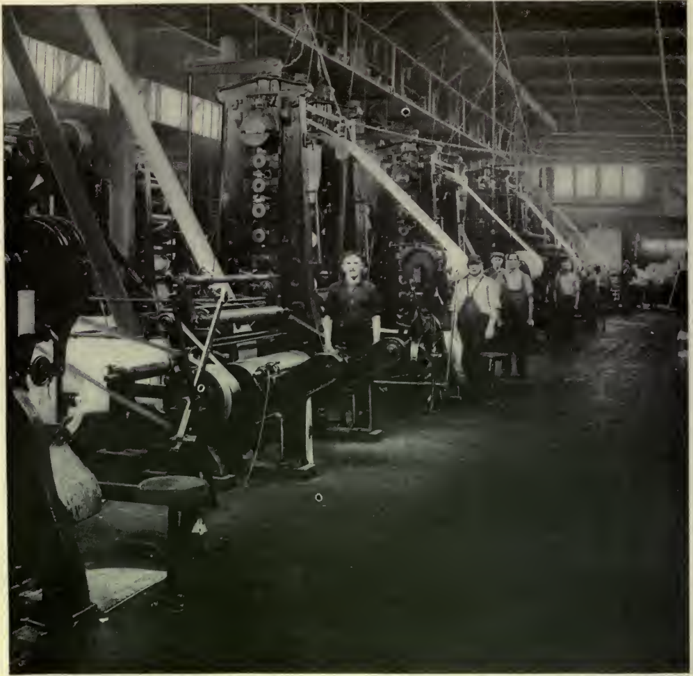
A BATTERY OF CALENDER PRESSES AT WORK FINISHING MAGAZINE PAPER
