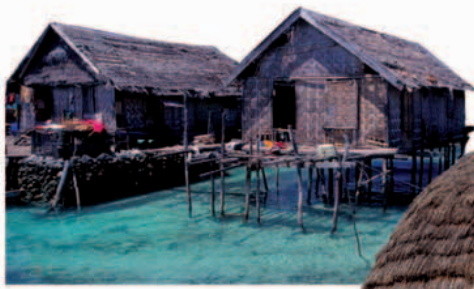
▲ STILT HOUSES Some people who live along coasts and rivers build their houses on stilts to avoid flooding.
