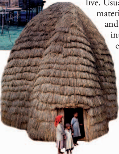
▶ BAMBOO HOUSES The Gamo people of Ethiopia make houses from split bamboo, which is woven and thatched.
