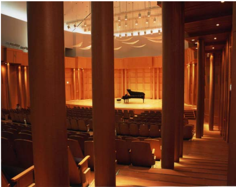
Photo 8.2 Tsuyama Music Cultural Hall with 52 columns each of 30 cm diameter around the walls
