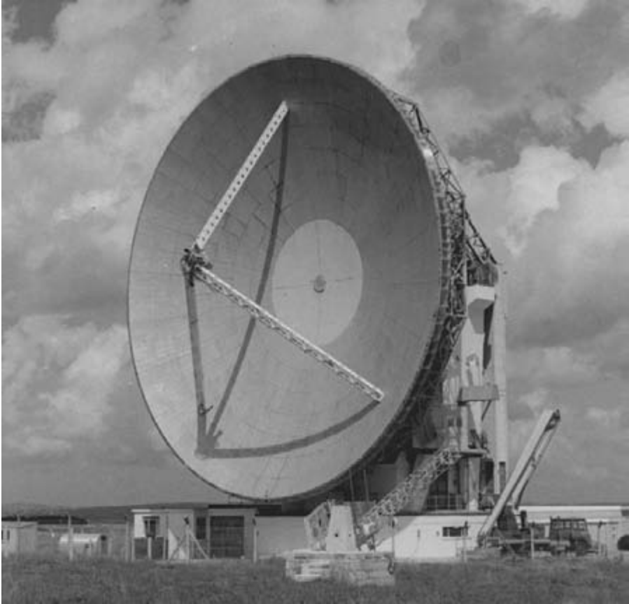
Figure 15.4 Post Office satellite communication ground station aerial No.1 at Goonhilly, Cornwall (1962)
