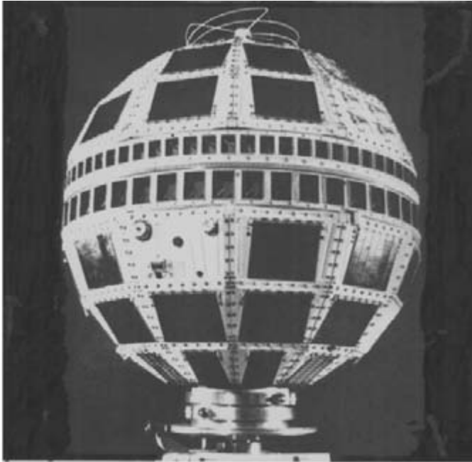
(a) ATT/BTL 'TELSTAR' Satellite (34.5 ins diameter, 170 lbs weight)
