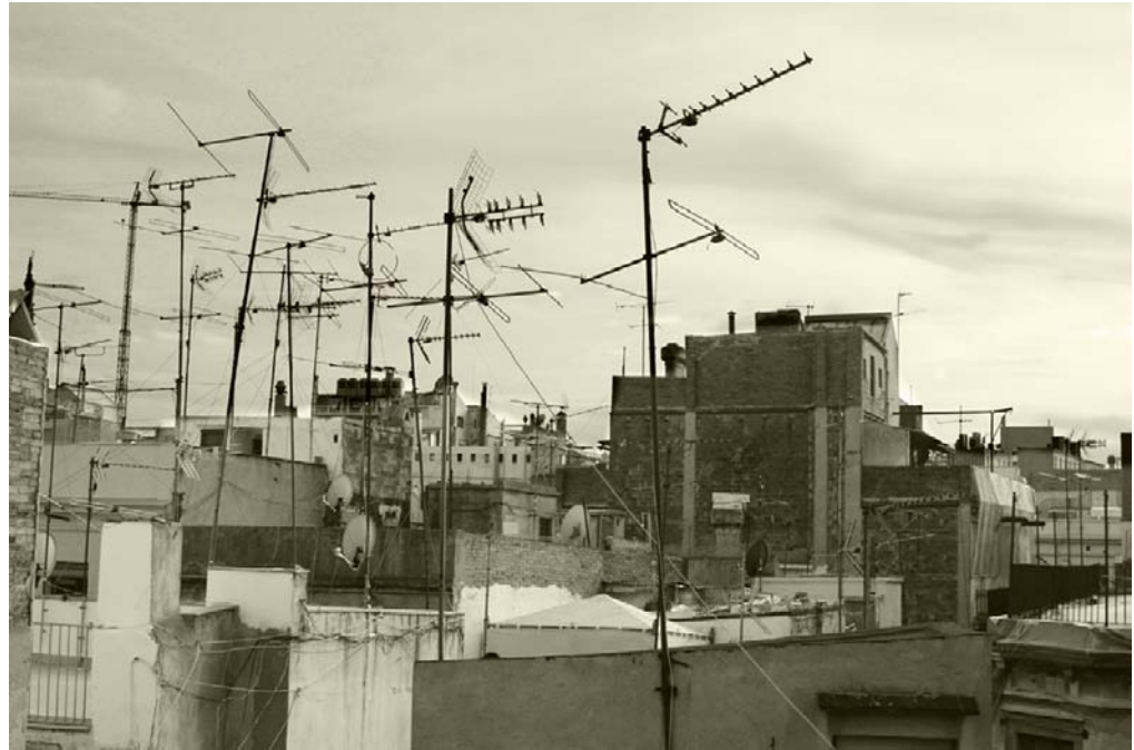
FIG. 4.1 These rooftops show an unsightly array of antennas and satellite dishes for receiving television and radio signals. This type of view is typical in major cities in the United States and developed countries throughout the world. The recent switch to digital broadcasting has actually increased the number of rooftop antennas. Photo courtesy iStockPhoto. ©dubassy, image #7418420.
