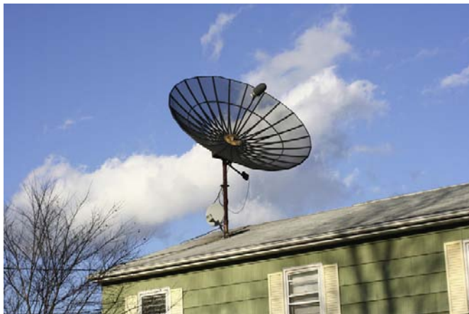
FIG. 4.2 This picture shows both an older C-band satellite receiving dish and a newer DBS dish mounted below it on the same mast. The DBS dish is about one tenth the size of the C-band dish above it. Photo courtesy iStockphoto. ©tomnackid, image #2687905.
