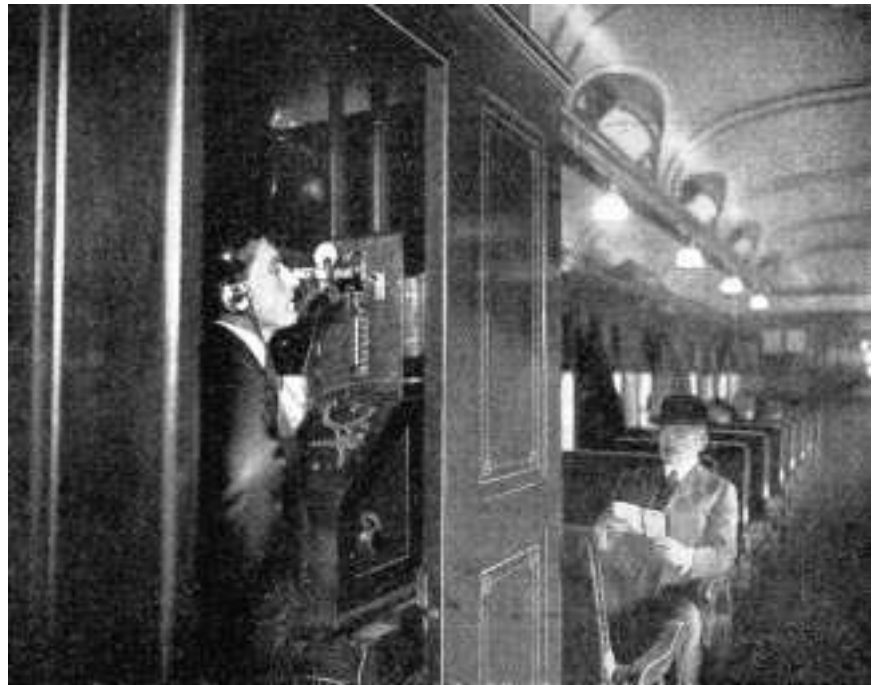
Fig. 14.2 Wireless telephony on the train. The installation is in a small cabin about 2 by 4 feet at one end of the car.
