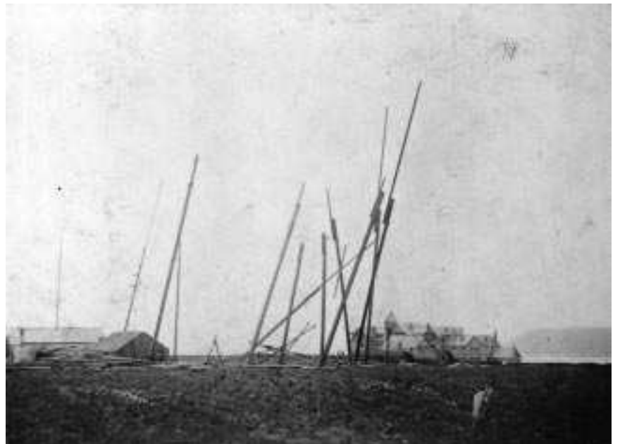
Fig. 6.7 (a) The aerial at Poldhu built for trans-Atlantic transmission. (b) Destroyed by a storm before it could be used.
