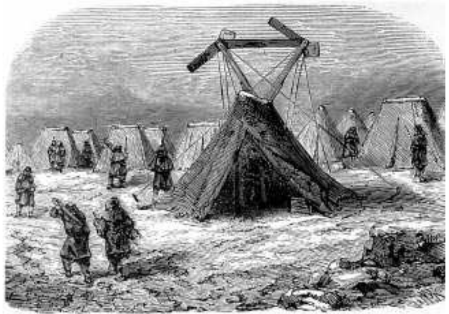
Fig. 3.6 The French mechanical telegraph in the Crimean War.
