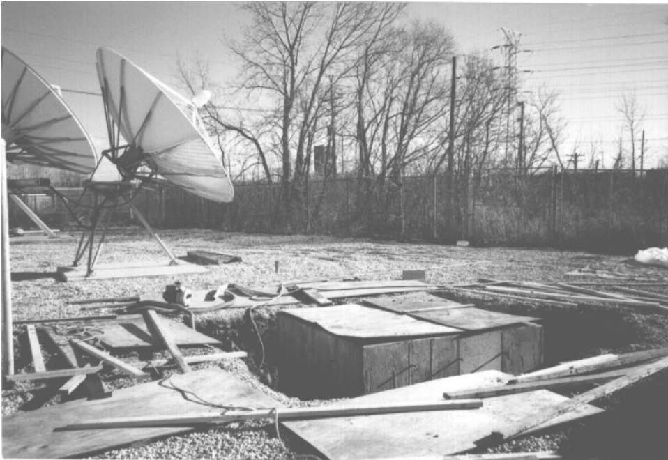
FIGURE 58.6 Antenna pad construction.
