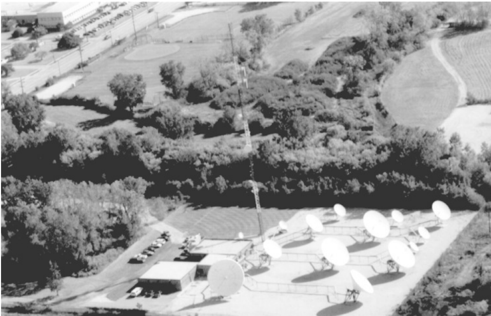
FIGURE 58.2 Teleport Chicago Earth station.
