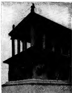
THE SOUTH WING, WEST AND SOUTH SIDES.
