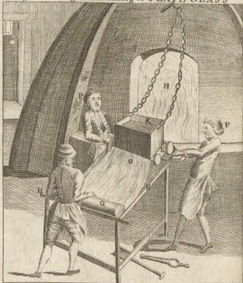
Fig. 2. Casting and Running of PLATE GLASS
